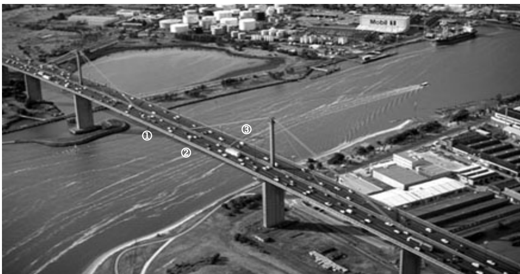
Figure 1 – View of the central steel spans of the Westgate Bridge, showing the approximate locations of three GPS receivers used in the monitoring study.
