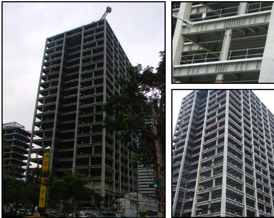
Figure 4-11 Xinyi District Commercial Building, Taipei, Taiwan
