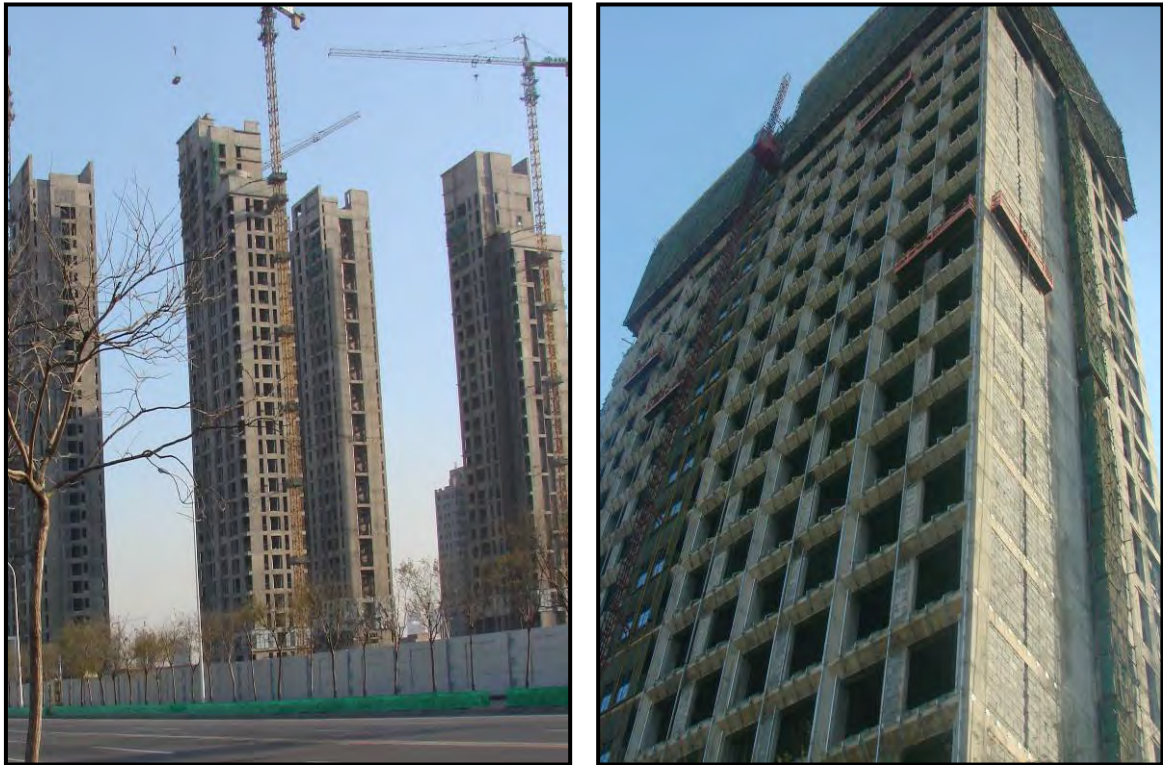
Figure 4-17 Tanggu Apartment, Tanggu District, Tianjin, P.R.China
