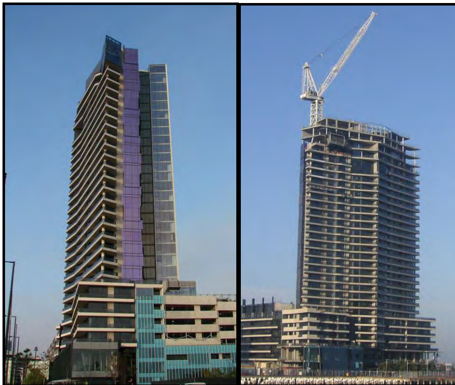
(a) Dock 5 in-use
