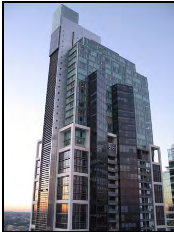
Figure 4-6 World Tower, Sydney, NSW
