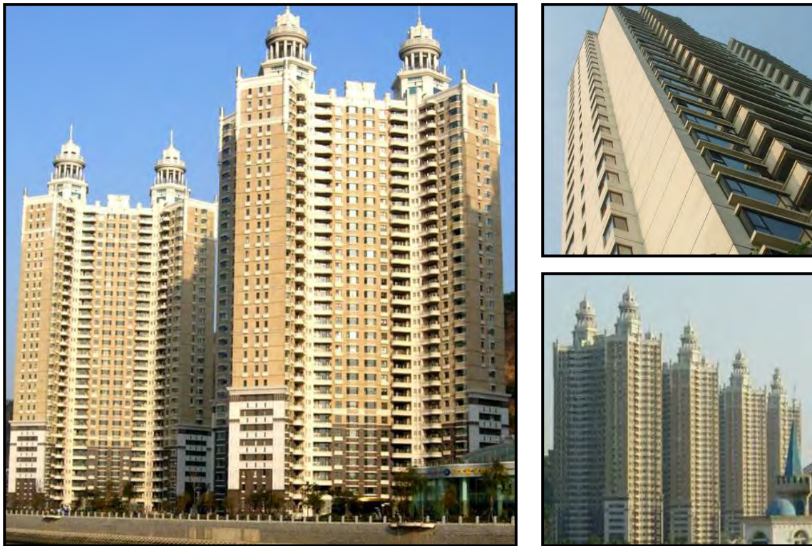
Figure 4-20 Xinghai Guobao Residential Building, Dalian, P.R.China
