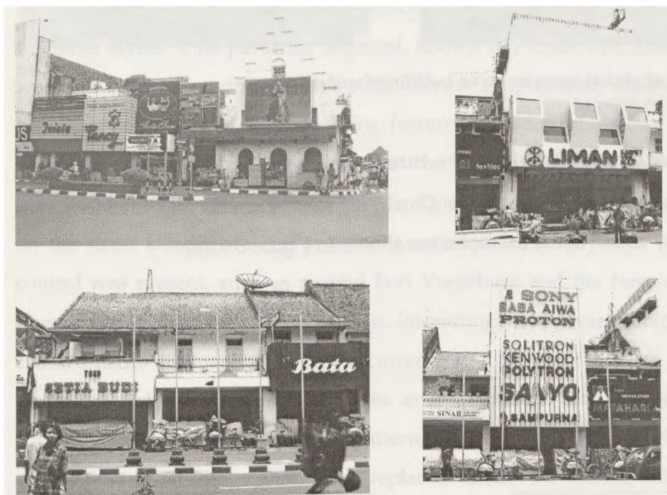
Figure 6. 39 Examples of the façade changes Source: Author's photographs.
