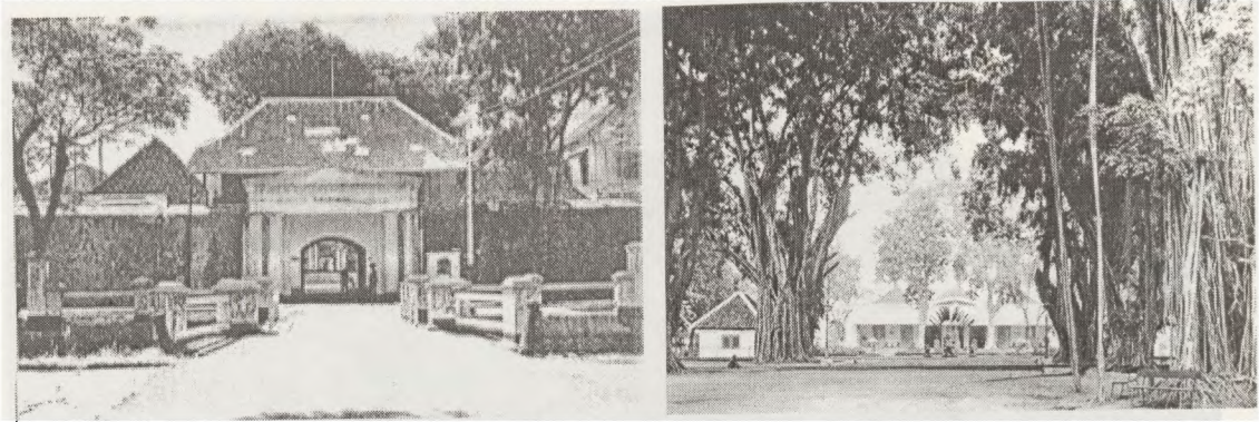
Figure 6. 8 Fort Vredenburg and Resident's House in 1830 Source: Buitenweg , 1965.
