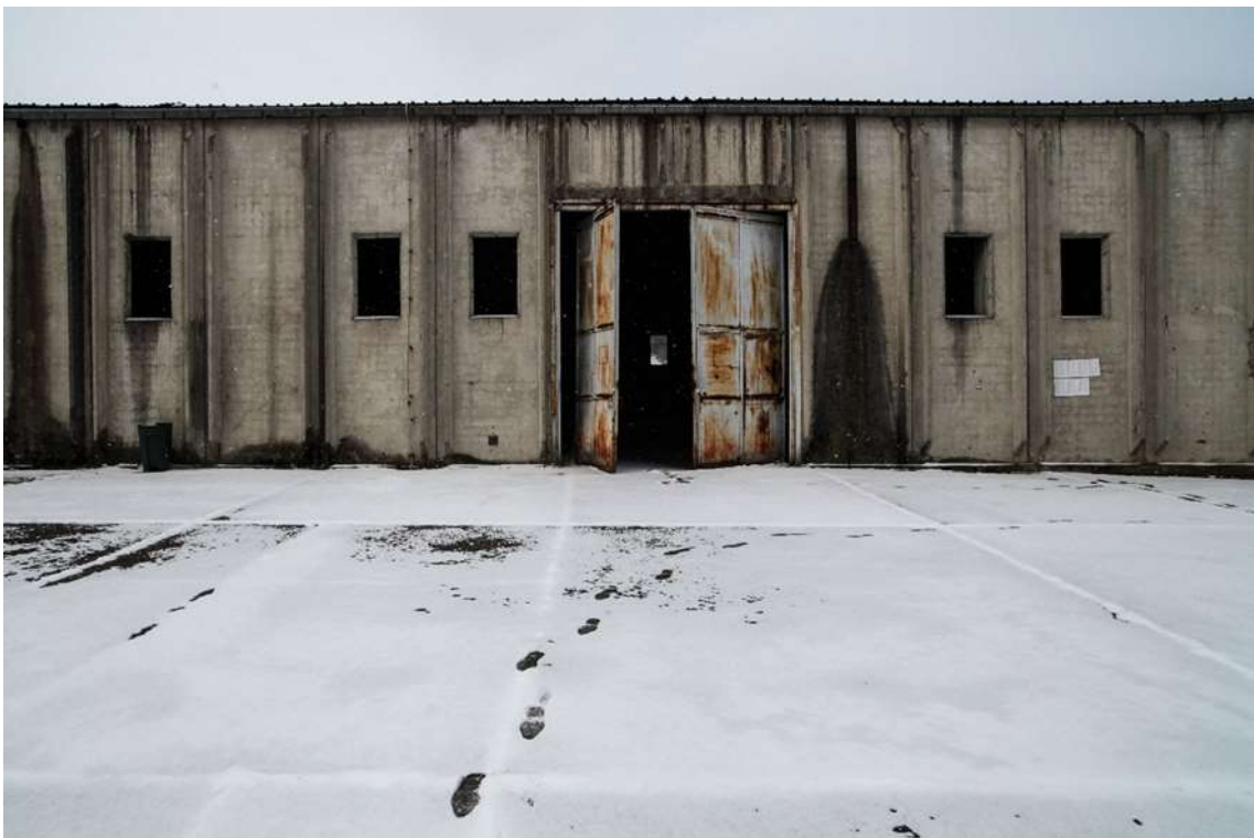
Figure 65. Elmedin Žunić, The battery factory , 2016.
