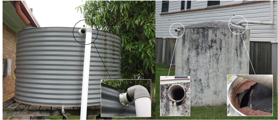
Fig 4. Non-compliant rainwater tanks (with anti-mosquito regulations) identified in Gin Gin containing Aedes aegypti . Inserts show detailed views of exposed overflows and rusted inflow sieves.
