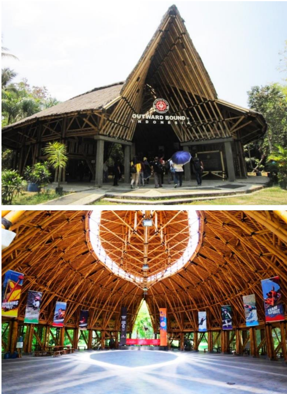
Figure 27. The Great Hall of Outward Bound Indonesia (OBI) Eco Campus shows contemporary use of bamboo in architecture Source: Andry Widyowijatnoko and Rakhmat F. Aditra, 2018 (reprinted with permission)
