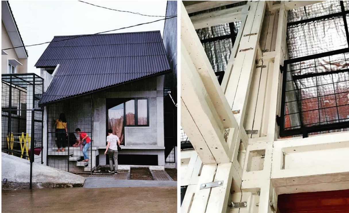
Figure 38. Hatika House (left) constructed using the RISHA structure (right)
