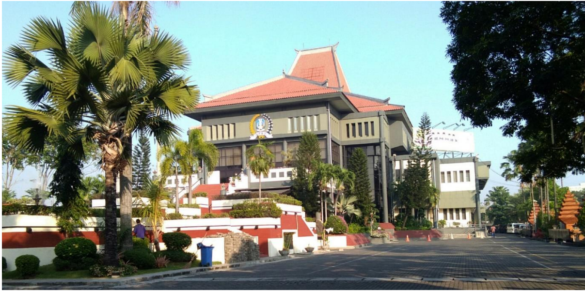
Figure 7. East Java's House of Representatives building
