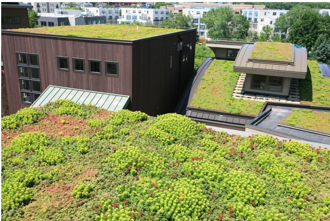
Figure 1.1. Shallow substrate extensive green roofs covered with succulents, in Milwaukee, Wisconsin, United States (source: liveroof.com ).
