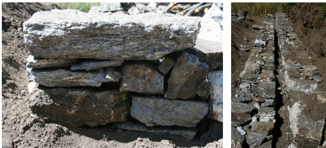
Figure 40 – Stone wall construction; inner and outer wall.
