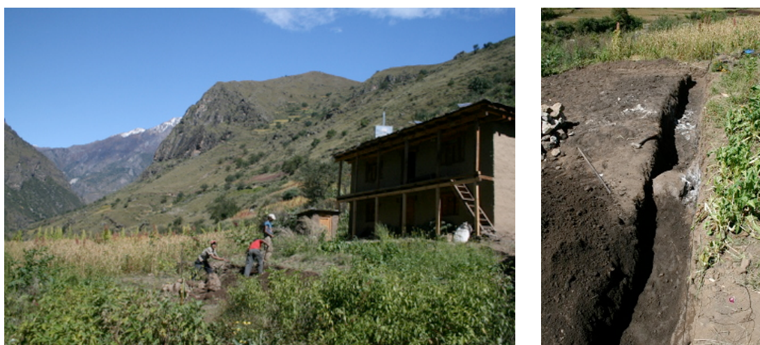
Figure 39 – Greenhouse site in Darapori village; excavating foundations.
