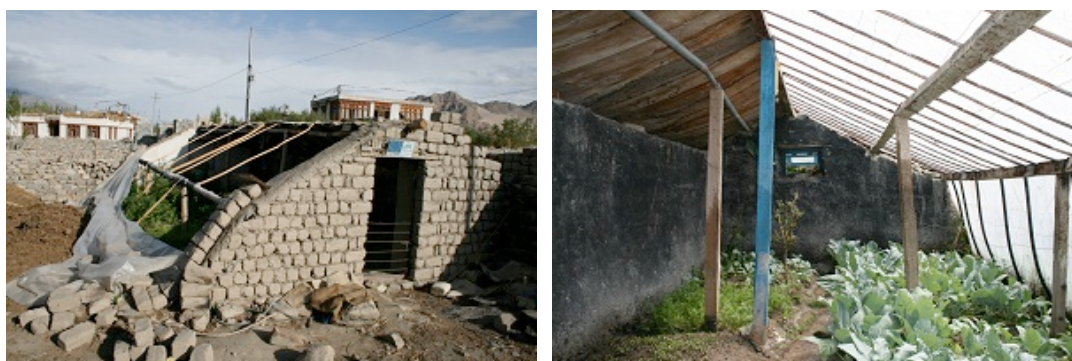
Figure 35 – Solar greenhouses in Ladakh (Photos – S Candy).
