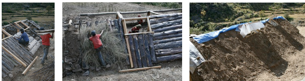
Figure 44 – Wooden planks on roof; adding straw layer; soil over plastic layer.
