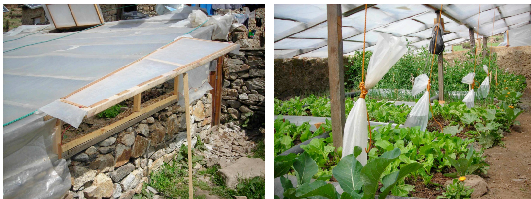
Figure 19 – Performance improvements for the HARS greenhouse (ventilation and water heat stores) (photos courtesy of R Fuller).
