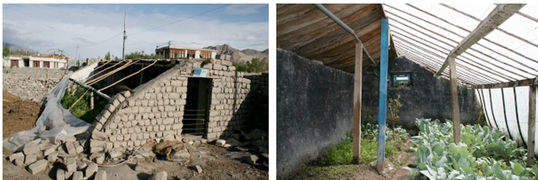
Figure 20 – Solar greenhouses in Ladakh (photos – S Candy).
