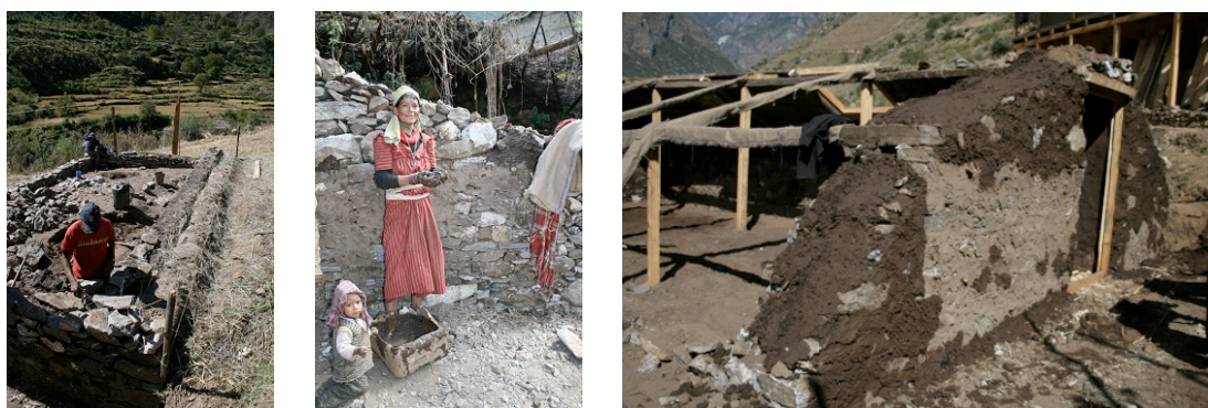
Figure 42 – Filling insulation in back wall; sealing walls with mud.
