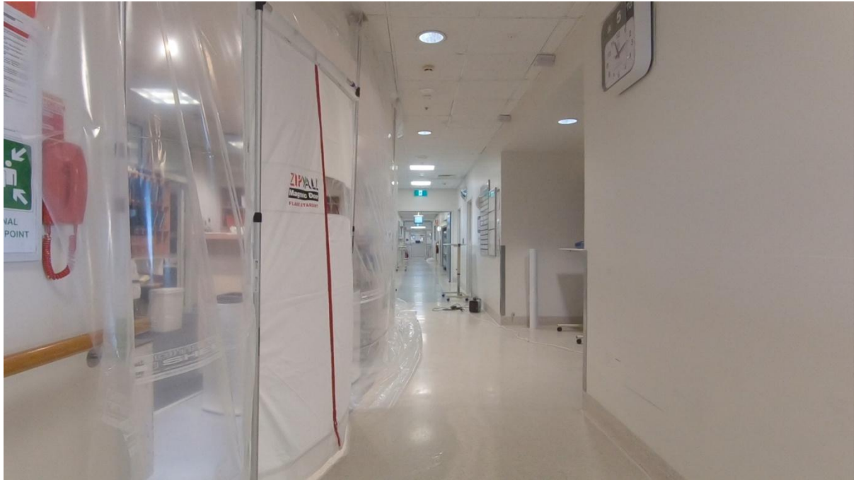
Figure S3: Photo of installed ZipWall™ at nurses' station
