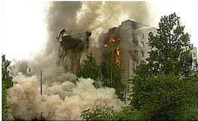
Figure 1.5: Collapse of a 9-storey building in Russia (Beitel and Iwankiw, 2008)
