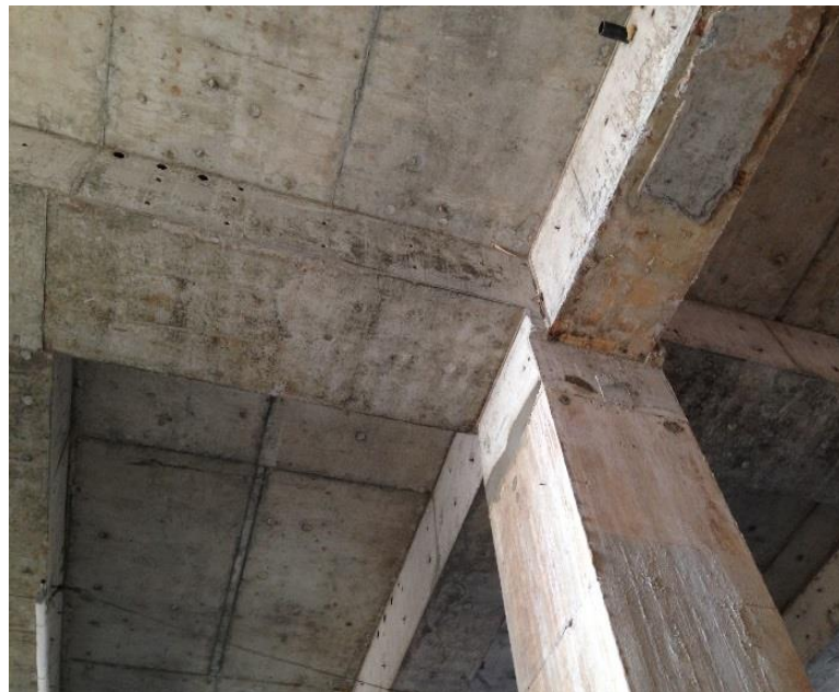
Figure 1.1: Conventional slabs supported by beams and columns
