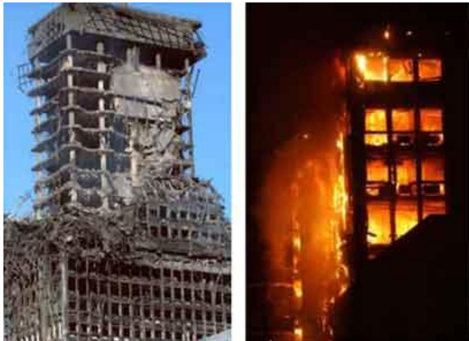
Figure 1.6: Partially collapsed building in Madrid, Spain due to fire (Hellenic Cement Industry Association, n.d.)
