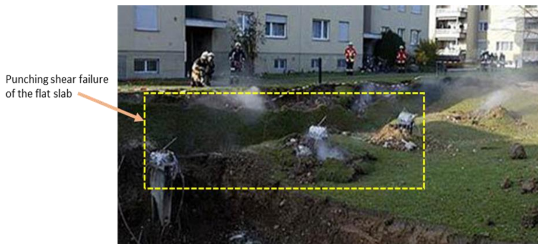
Figure 1.7: Underground car park collapse in Gretzenbach, Switzerland in 2004 (Michael Noblett, n.d.)
