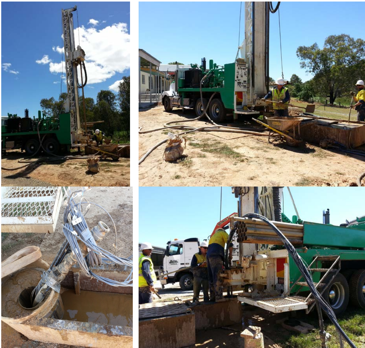
Figure B-56: Drilling and installation of instrumented ground loops
