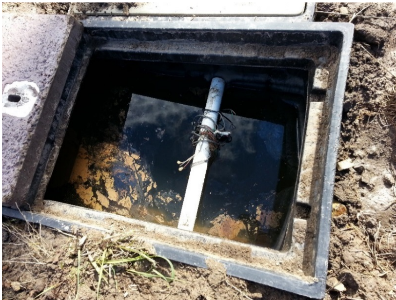
Figure 3-13: Waterlogged pit in Murrindindi due to consecutive period of heavy rainfall
