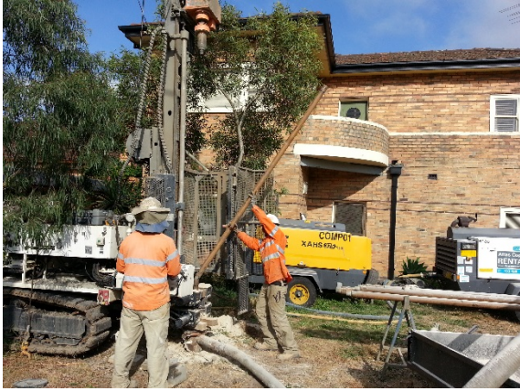
Drilling of a vertical GHE at Thornbury
