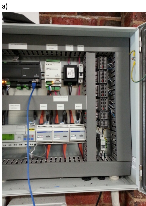
Figure 3-8: Standard data logger used in the SEPD project from (a) Emerson™ and (b) Phasefale™
