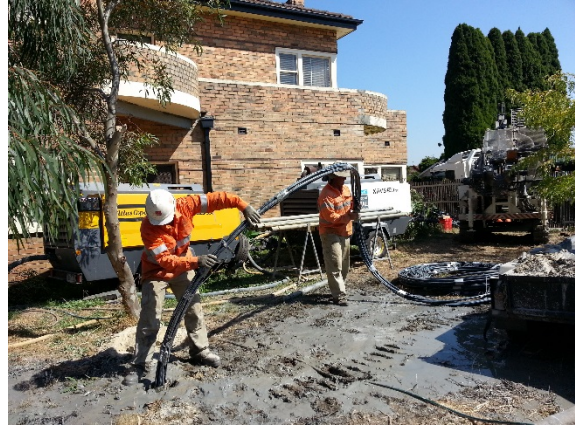
Vertical GHE installation at Thornbury
