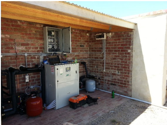
GSHP and data logger at Kangaroo Ground 2
