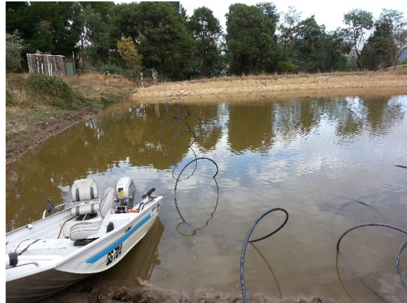
Installation of pond loops at Murrindindi
