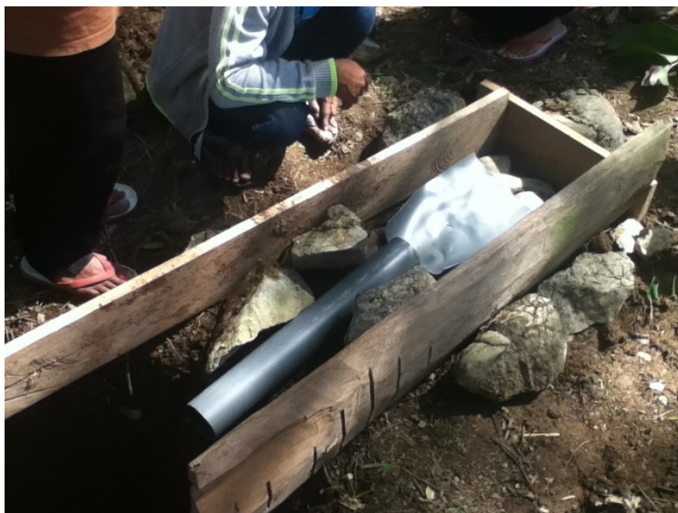
Figure 6-5 'Home-made' mould with pipe, Community A (Photo: Naomi Francis)
