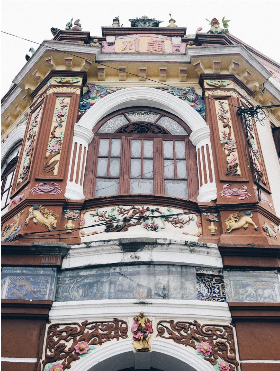
Figure 48. An ornate corner shophouse in Kuala Pilah, featuring a combination of Chinese and western ornamental features executed in plaster and cut porcelain work. Photograph by the author.
