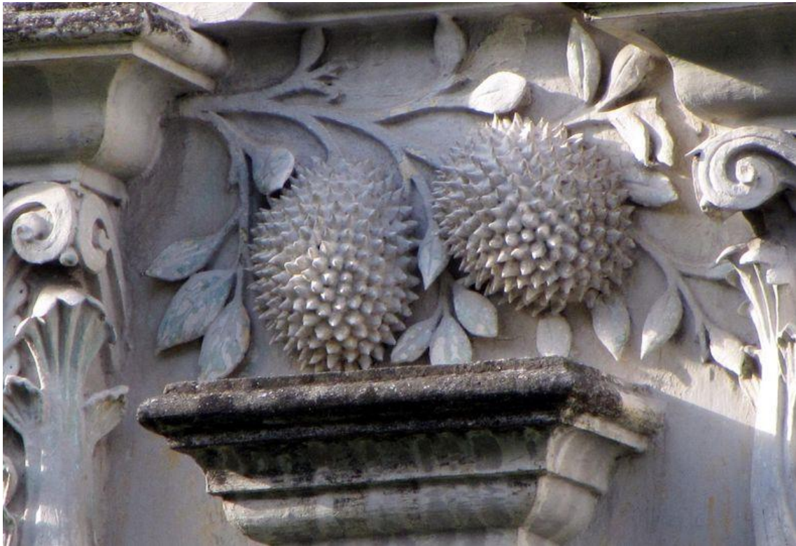
Figure 43. Ornamental plaster durians sit atop a Doric capital in an early twentieth-century bungalow on Macalister Road, Penang. Mark Lay.
