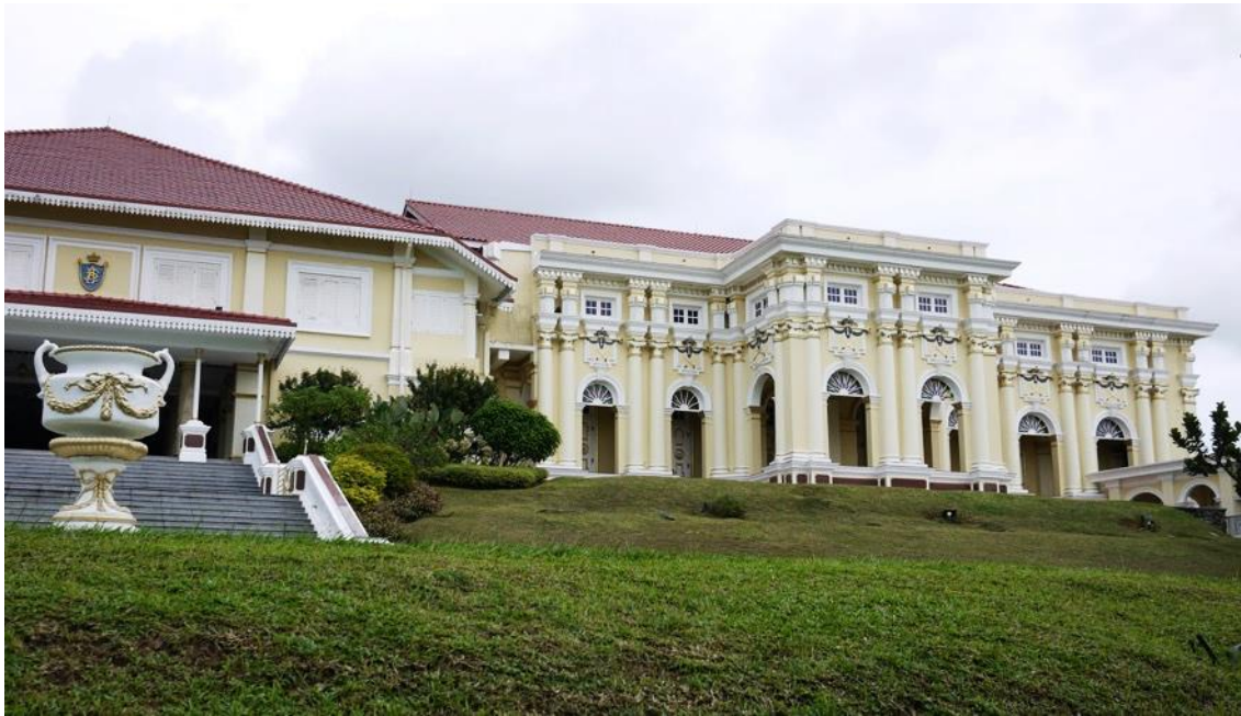
Figure 27. Southern elevation of the Banqueting Hall at the Istana Besar. Photograph by the author.
