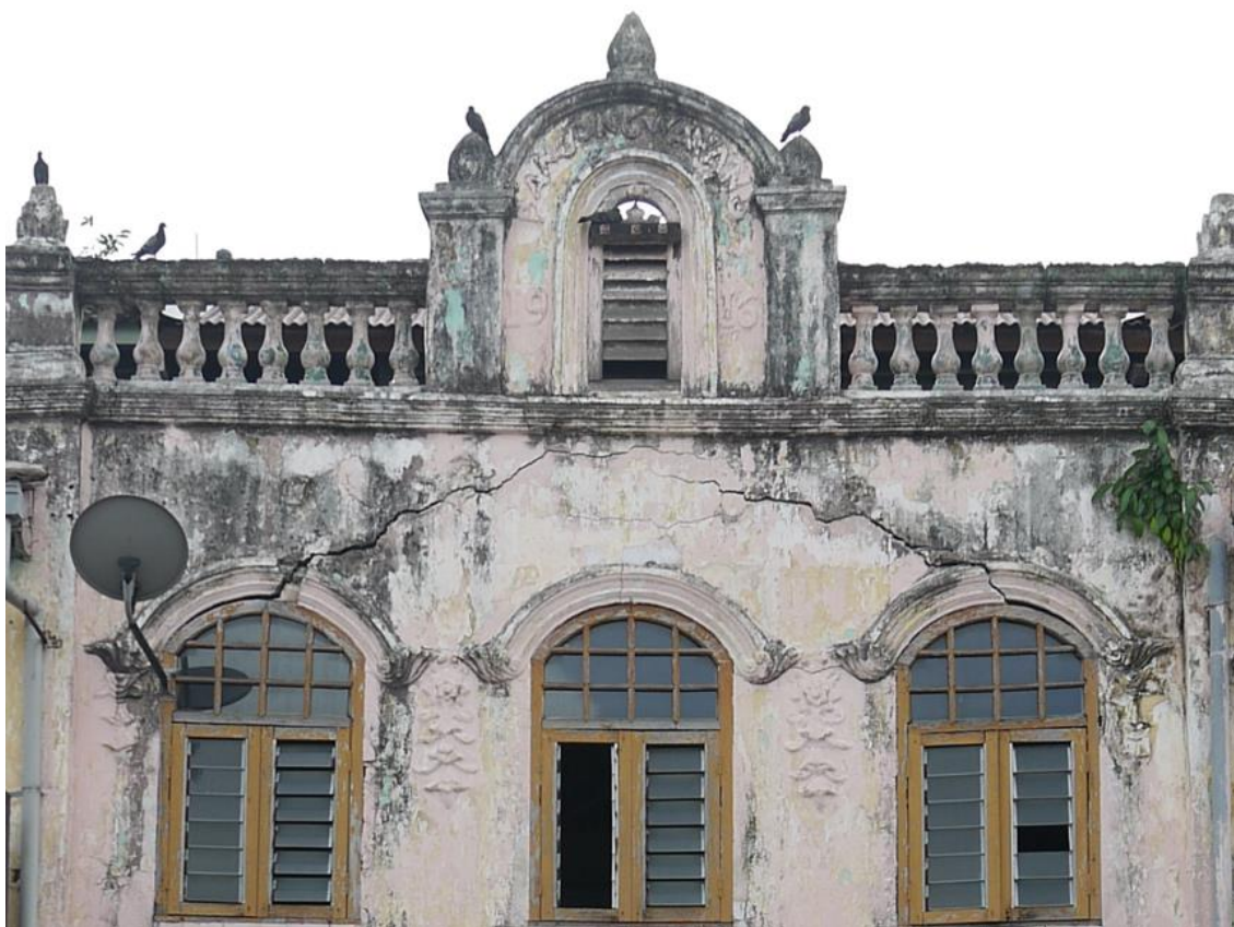
Figure 69. Façade details of a former theatre dated 1916 in Kuala Pilah. Photograph by the author.
