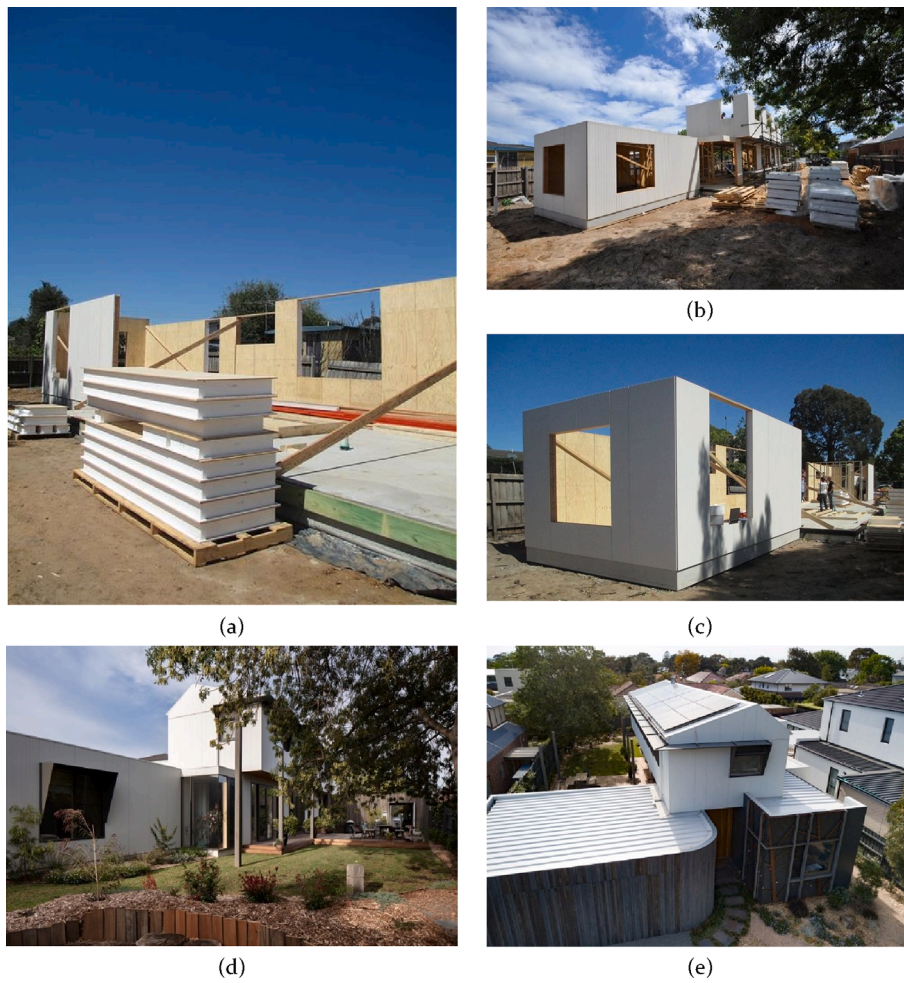
Fig. A3. The images of the selected building located in Melbourne, Australia: (a), (b), (c) under construction and (d), (e) completed [52].
