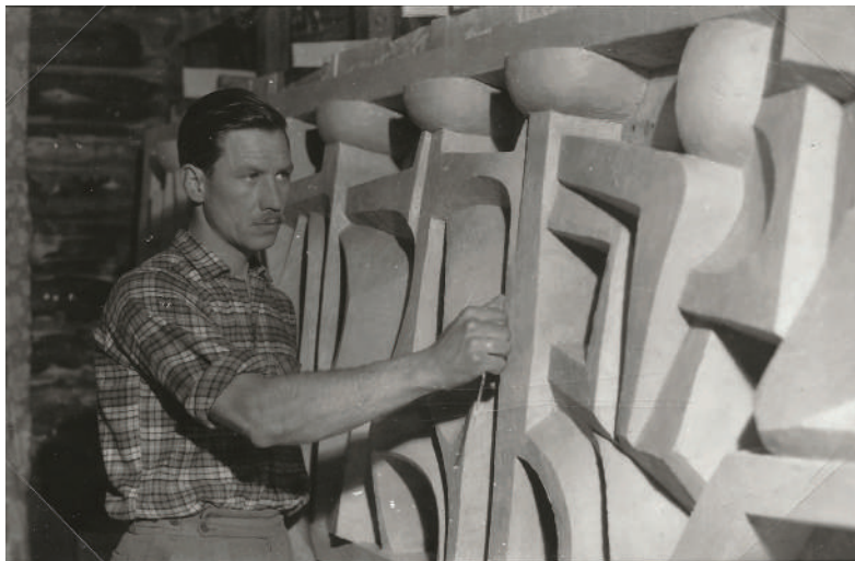
14, Zikaras working on the cast concrete Union House Panels for the University of Melbourne, 1957–1958, photo Mark Strzic courtesy artist's estate, Melbourne
