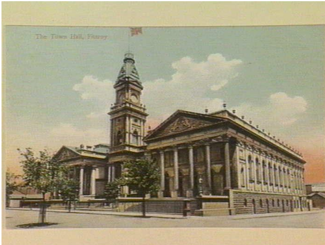
The Fitzroy Town Hall complex c. 1906 State Library Victoria, H90.160/991.
