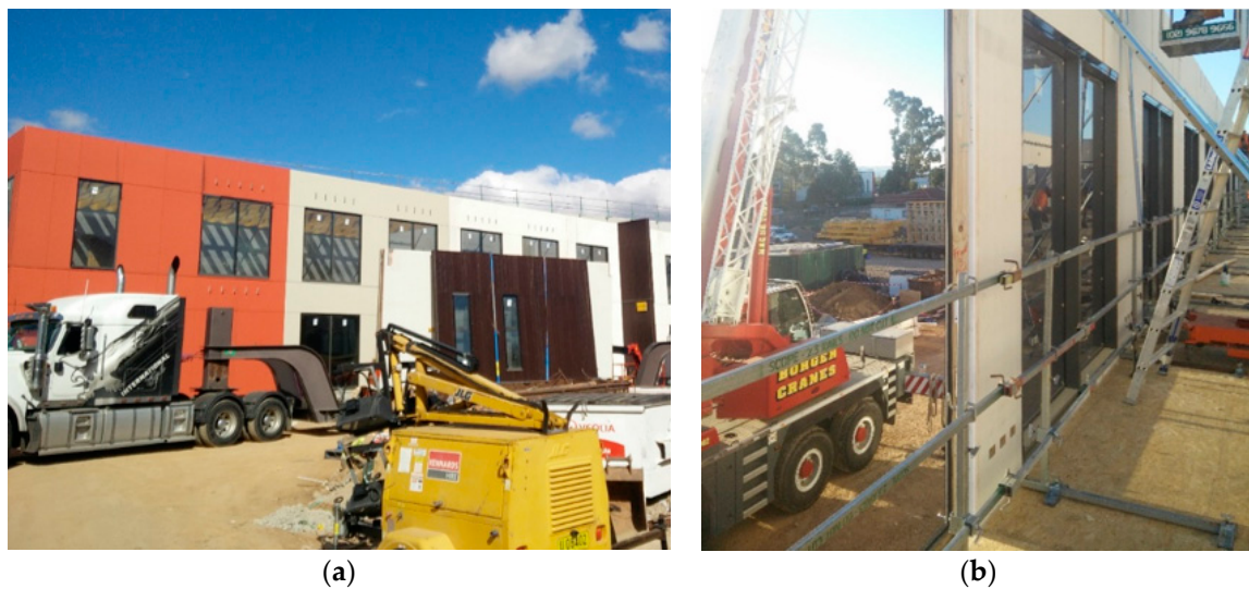
Figure 16. Implementation with panelised form of prefabricated construction: (a) Commercial office building using the gasket seals; (b) EPDM gasket seal positions on the wall towards the outside face.
