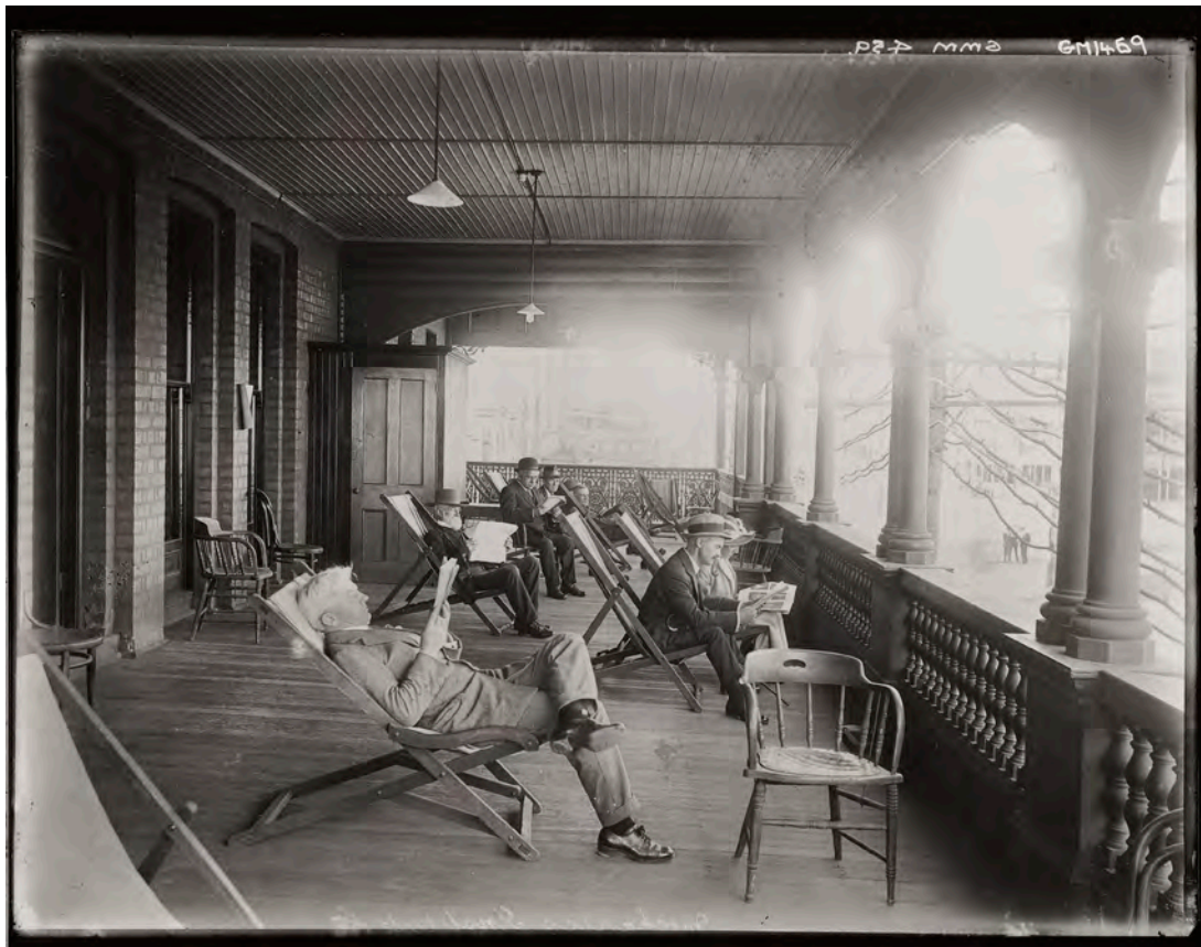
Figure 4.29: The balcony of the Kalgoorlie Mechanic's Institute
