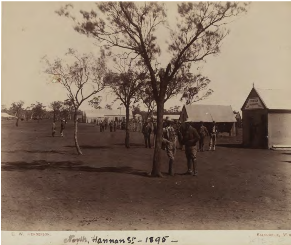
Figure 4.6: North Hannan Street 1894/5
