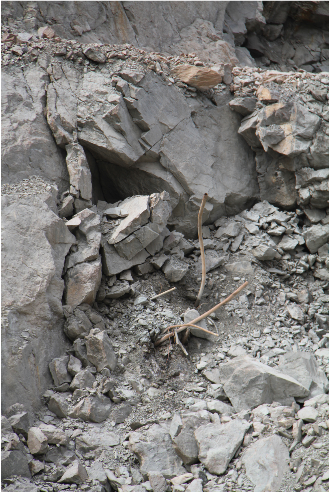
Figure 1.5: Detail of tunnel opening where the open cut mining has exposed the infrastructure of the tunnels, and 'drives' of underground mining. Photograph by the author
