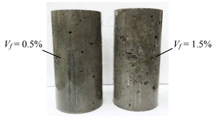
Figure 4 Comparison of air voids on the surface of typical samples with volume of 0.5% and 1.5% steel fibres
