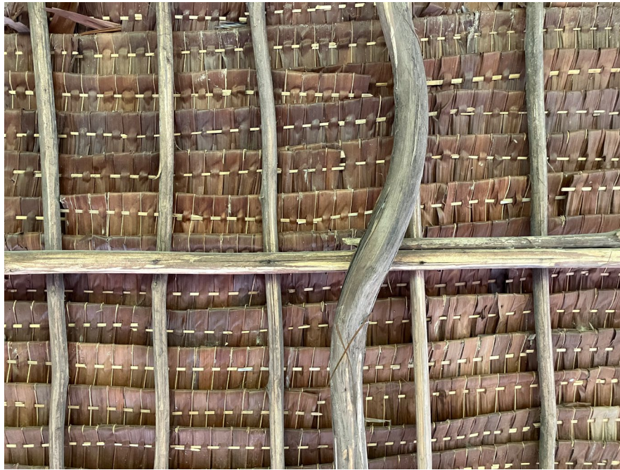
FIGURE 3 | Natangura roofing made from woven palm leaves. Source: Sebastian Salay.
