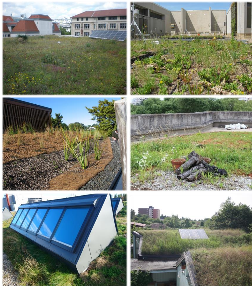
Figure 1.1 Green roofs adorn urban landscapes worldwide, symbolising the expansive reach of this sustainable practice in global green infrastructure. Featured locations, clockwise from top left: Ludwigsburg, Germany (Christine Thuring); Texas A&M University, USA (Bruce Dvorak); Chiba University, Japan (Ayako Nagase); Hanover, Germany (Chiara Catalano); Umeå, Sweden (Joel Lönnqvist); Auckland, New Zealand (Robyn Simcock).
