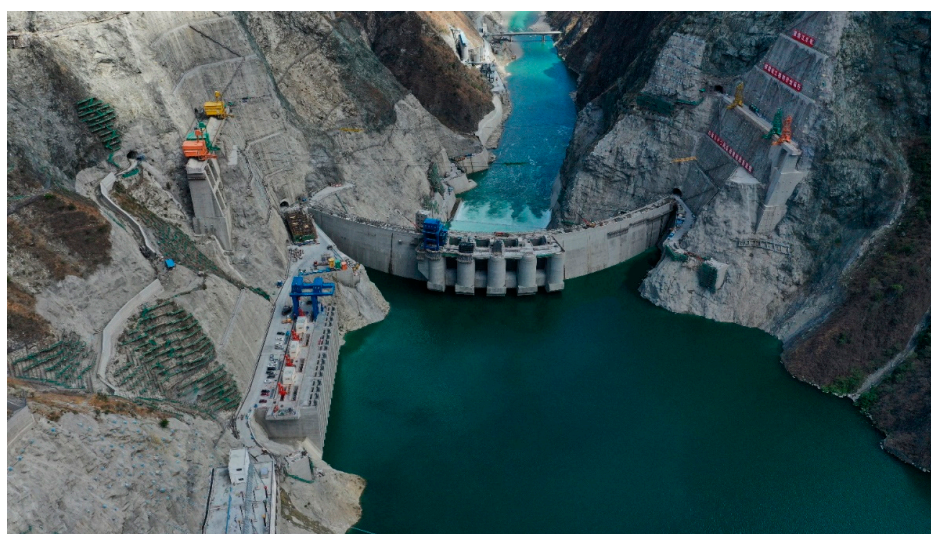
Figure 7. The Yangfanggou hydropower project.
