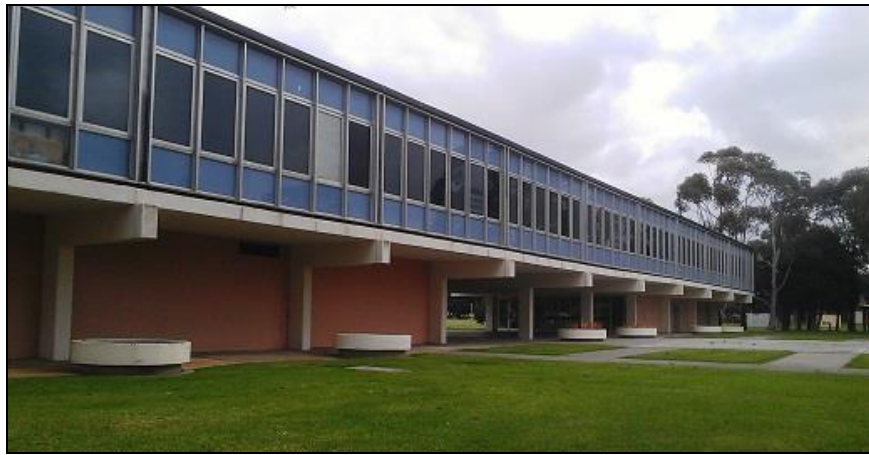
Figure 66: RAAF Academy library building, Point Cook (S. Campbell-Wright)
