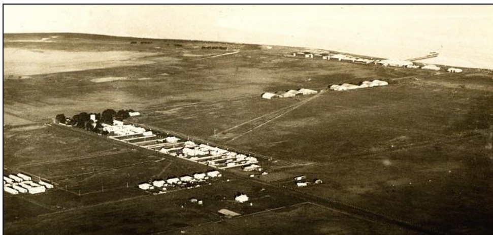
Figure 50: Point Cook RAAF base looking south-east (RAAF Museum, Point Cook, PCK Base box file)
