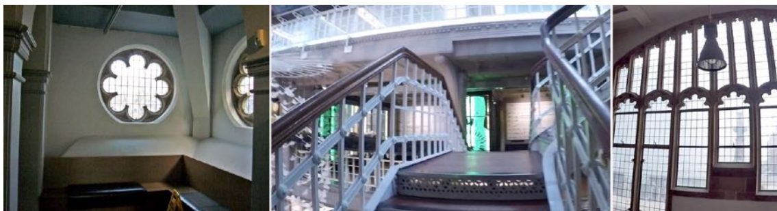
Figure 27. a. Rose windows / b. Stairs between levels / c. Neo-Gothic windows
