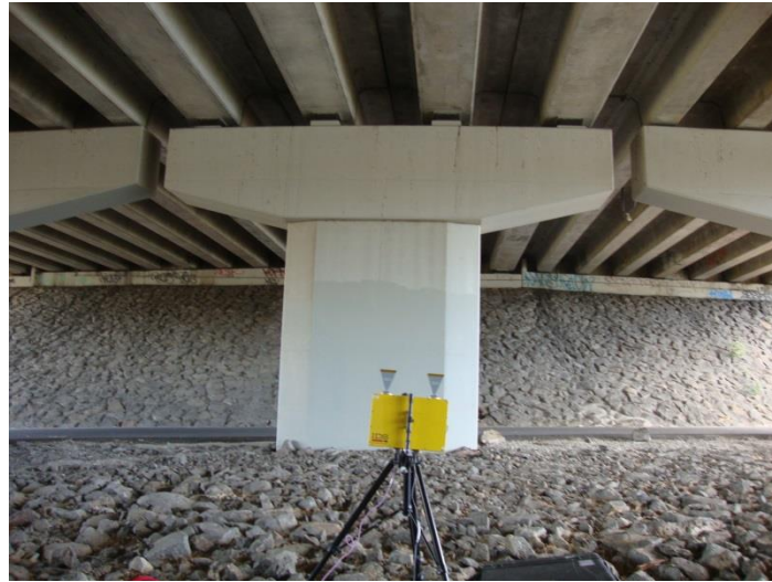
(a) View of Merlynston Creek Bridge during the in-field test using non-contact sensors IBIS-S
