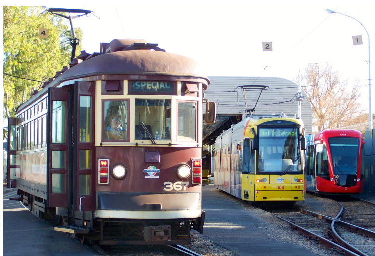
Figure 7.1: Tram depot in Adelaide, South Australia. Source: https://bit.ly/3d24m54 (© SCHolar44, 2018, original by © Adelaide h class, 2009, public domain).
