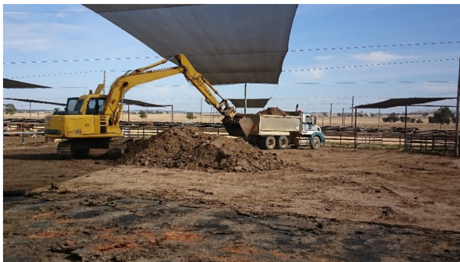
Figure 4. 3 Cleaning and removal of manure from cattle pens: excavator (yellow equipment) used for scraping and loading manure into truck.
