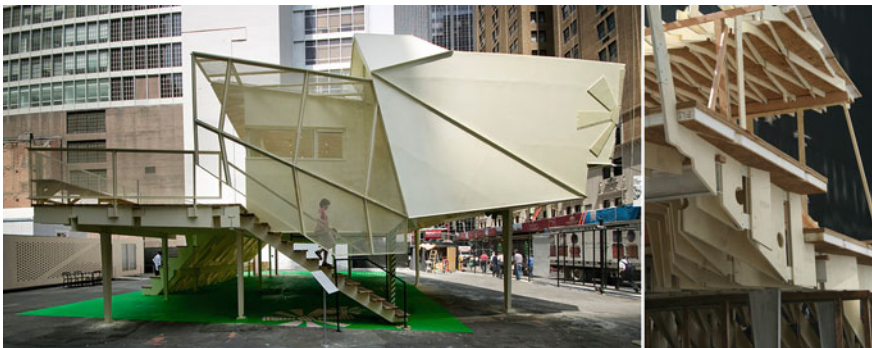
Fig. 3 ‘Burst*008’ at the MoMA Exhibition 2008. On the left, end elevation view. On the right, oblique view of the frame. Source Gauthier Architects archive [online]. Available at: http://gauthierarchitects.com/work
