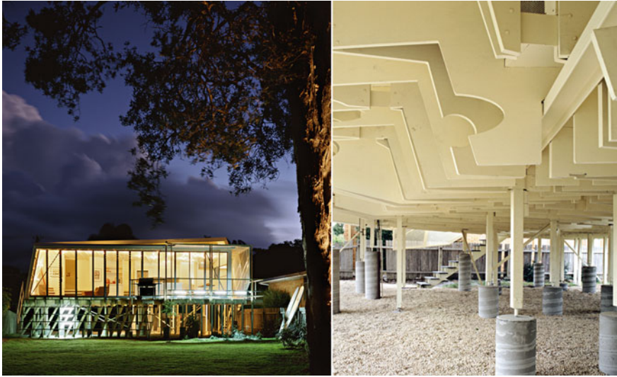
Fig. 2 ‘Burst*003’, 2005, on the east coast of Australia: on the left, the view from the rear yard. On the right, view of the undercroft, where the structural system is fully visible. Source Gauthier Architects archive [online]. Available at: http://gauthierarchitects.com/work
