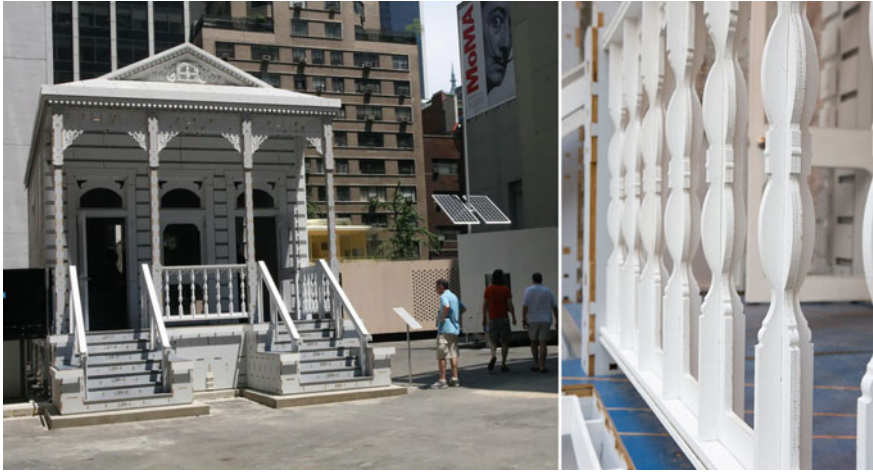
Fig. 7 The ‘Digitally Fabricated House’ for New Orleans at the MoMA Exhibition 2008: front view and details of the CNC components of the balustrade. Source Professor Lawrence Sass, photo by Suzanne Camarata Ball
