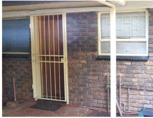
Figure 6.2 Security grills on the front door and window of a suburban home.
