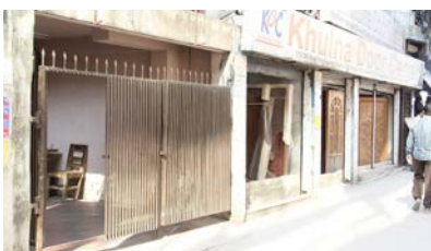
E: 152/2/M, Green Road Fig. 8.18: Building 18
