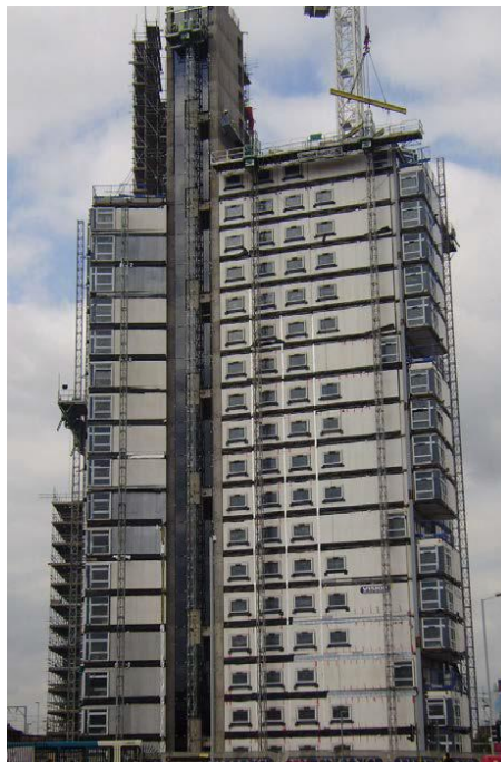
Figure 2-53 A 25-storey modular building in Wolverhampton, UK [2]
