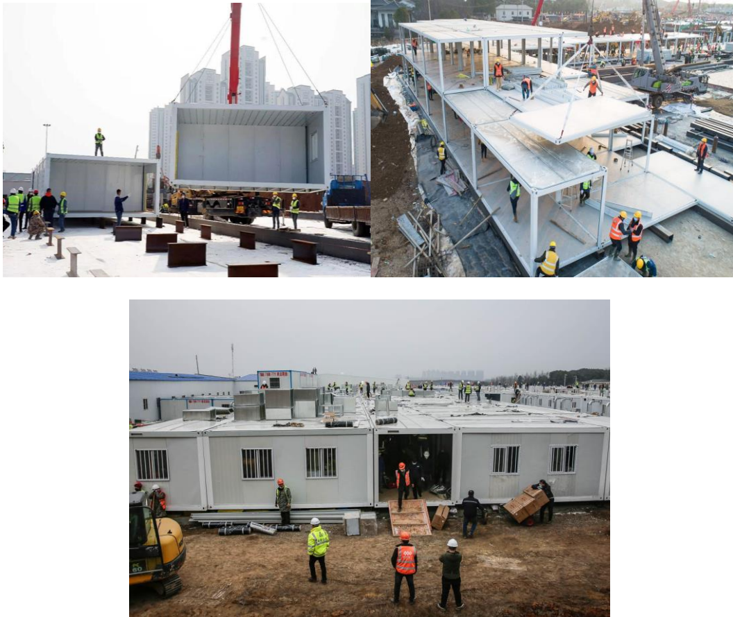
Figure 1-2 Wuhan, China, hospital construction, which was completed in 10 days
