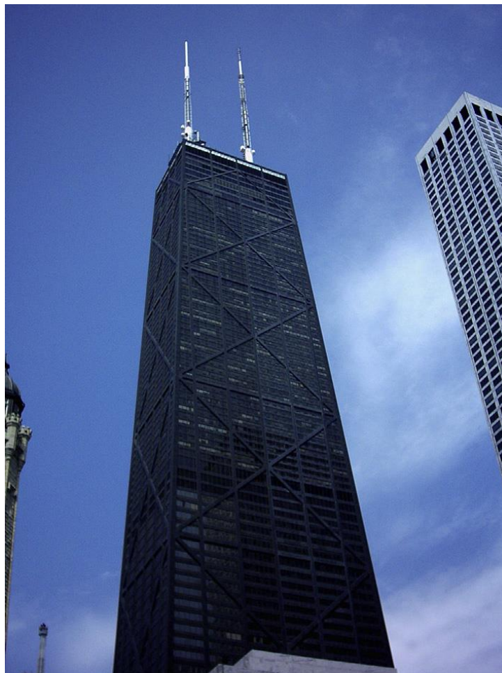
Figure 2-45 Braced-tube structural system incorporated building (John Hancock Centre in Chicago, USA) [2]
