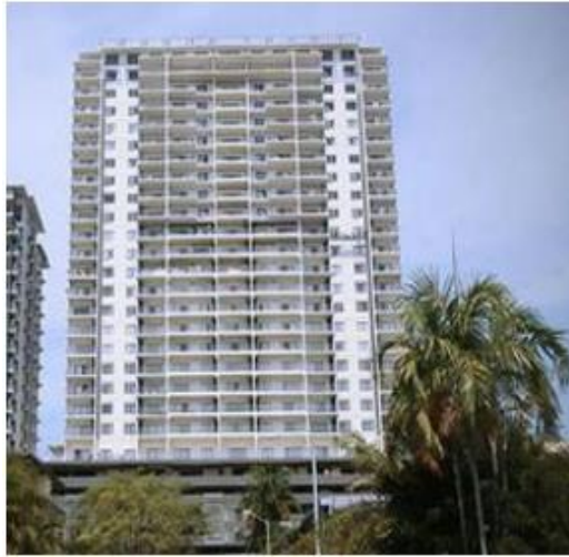
Figure 1-5 SOHO apartment building, Darwin, Australia [12]
