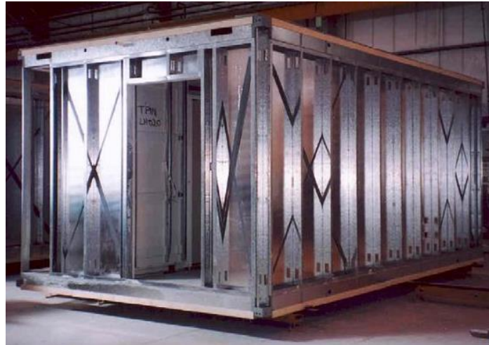
Figure 2-5 A typical load-bearing module [1]
