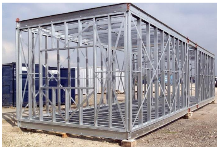
Figure 2-6 A corner-supported module [2]
