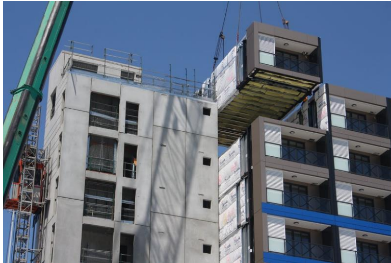
Figure 2-52 One9 Apartments, Melbourne, Australia [12]
