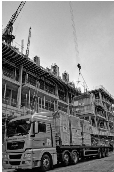
Figure 2-4 Installing bathroom pods in a concrete framed building [2]
