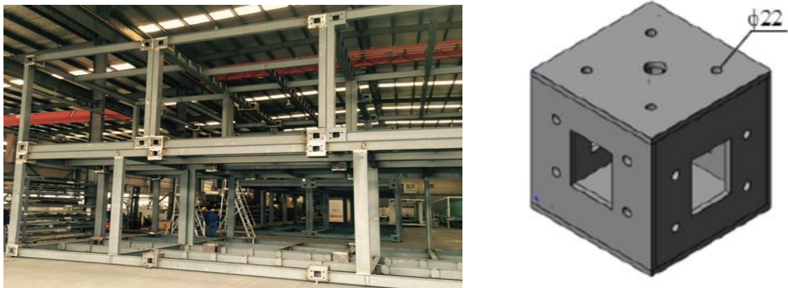
Figure 2-19 Steel bracket connection introduced by Doh et al. [41]
