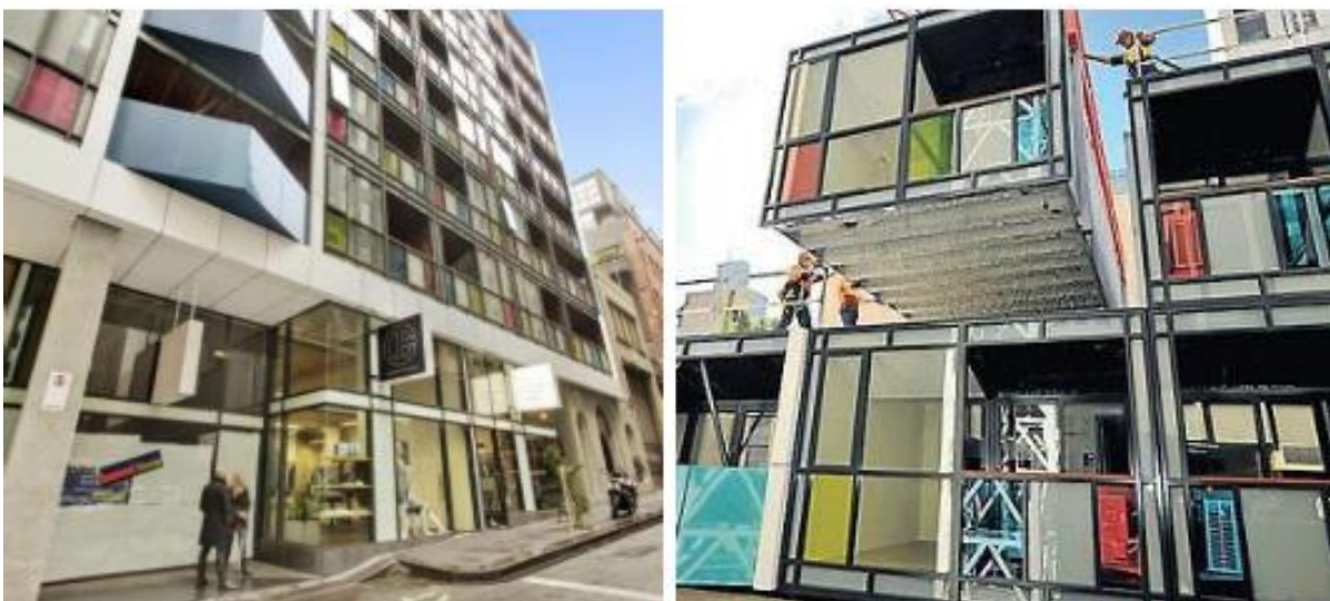
Figure 1-4 Little Hero building, Melbourne, Australia-8 storeys, 58 modules [12]
