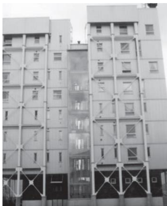
Figure 2-56 Modular units used in a tubular framework in Tampere, Finland [67]
