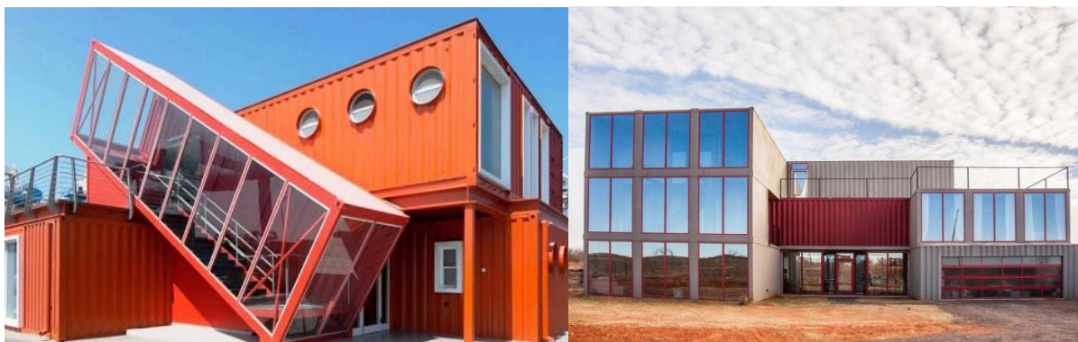
Figure 2-2 Shipping containers used for residential and commercial purposes
