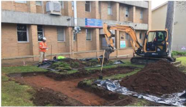
July 2019 works on-site
