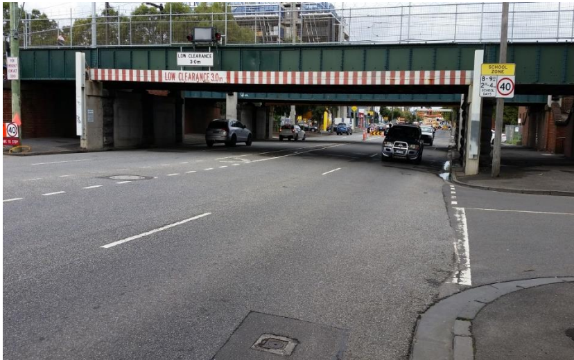
Figure 4.2: Montague Street Bridge in South Melbourne, Australia
