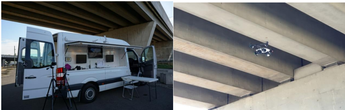
Figure 2.1: Unmanned aerial vehicle-based automatic bridge inspection and data acquisition
