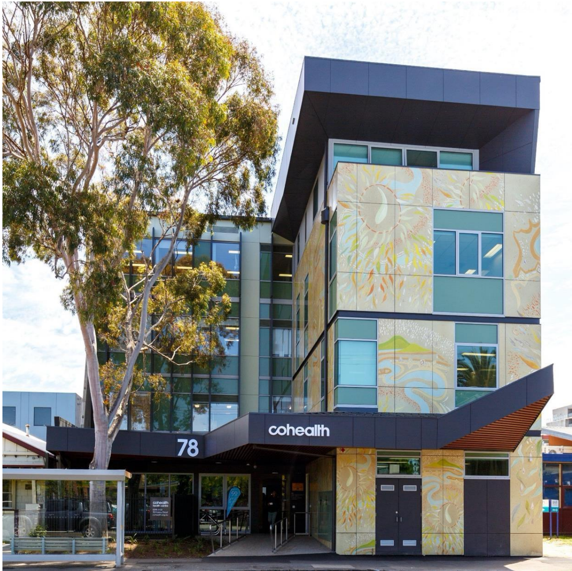
Fig. 12: Ngardarb Francine Riches (Bardi/Jawi, Karajarri) and Tony Riches. Exterior view of the CoHealth Building. 2016. Digital Photograph. 16.48 x 16.48cm.
