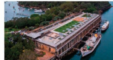
Precedent: Waverton Coal Loader, Hassell and North Sydney Council (2005-08) Photographs: Nathaniel Hughes, Copyright, North Sydney Council (2008)
