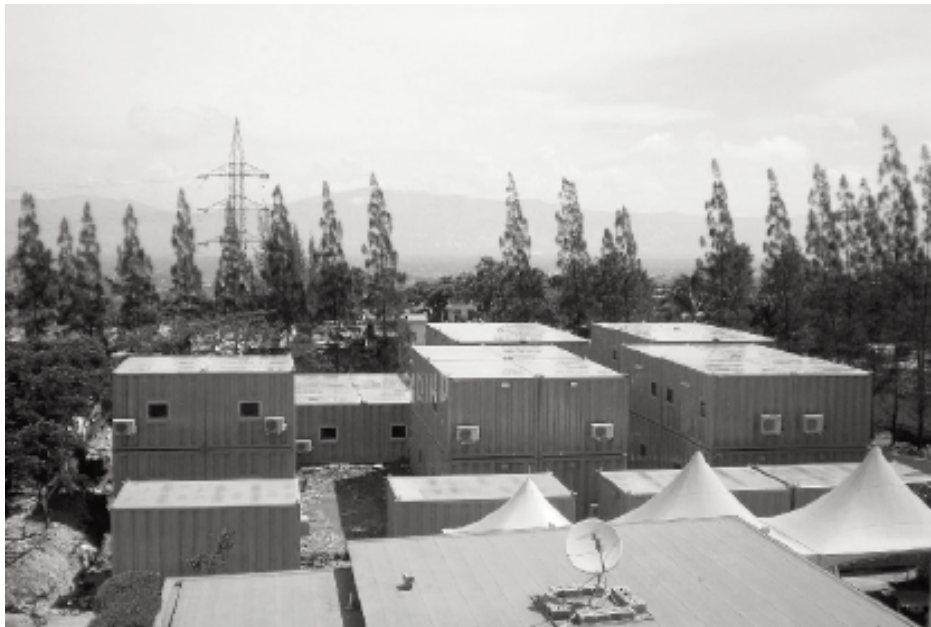
Figure 6. Modular housing units installed by the Canadian Embassy in Haiti (source: Sullivan Land Services, 2010).
