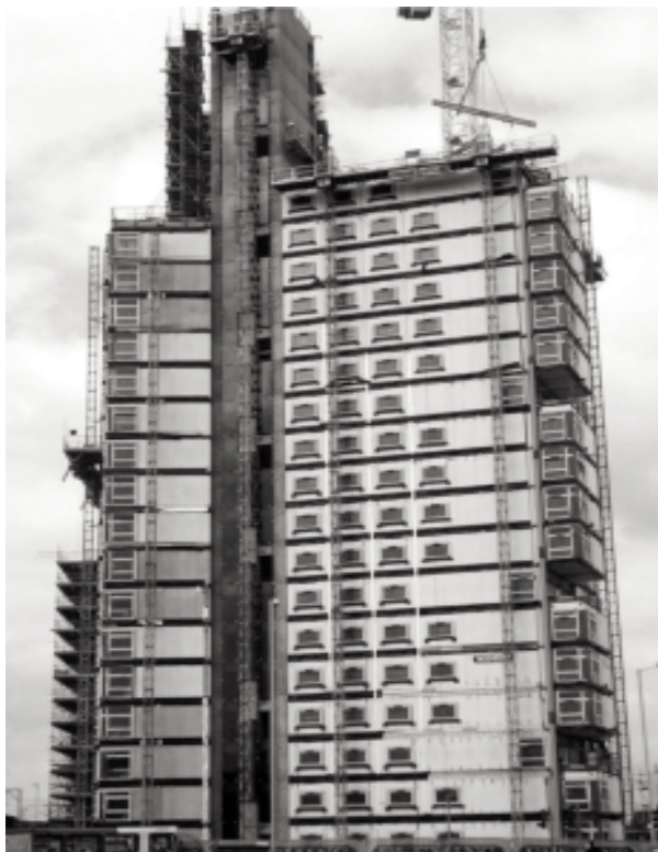
Figure 4. 25-storey student housing building in Wolverhampton, UK (source: Lawson et al, 2012).
