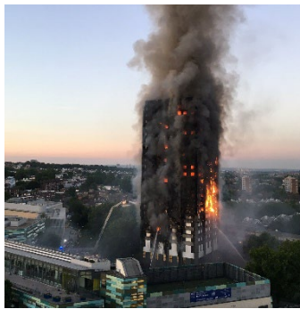
Figure 1: Recent example of combustible facade fires in Grenfell Tower, London, UK on 14 June 2017.
