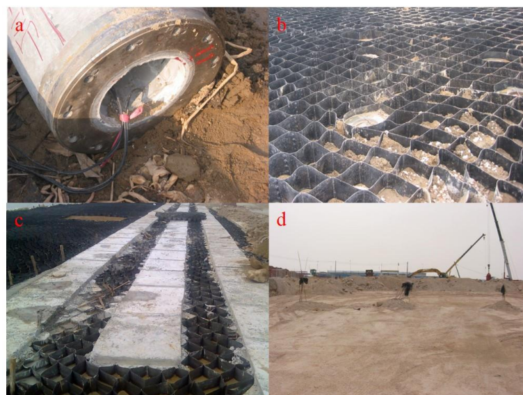
Figure 5. The steps used to install monitoring sensors in the riverbank slope: (a) sensor calibration; (b) geocell and anti-slide pile layout; (c) grouting and sealing; (d) filling.
