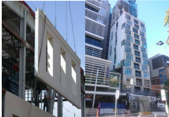
Figure 2.4. Prefabricated precast concrete cladding panel [9]
