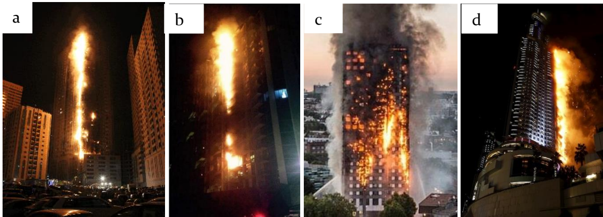
Figure 2.7. Façade fire: a) Al Tyer tower fire in Sharjah, 2012; b) Lacross building fire in Melbourne, 2014; c) Grenfell tower fire in London, 2017; d) Torch tower fire in Dubai, 2015, 2017 [23-26]
