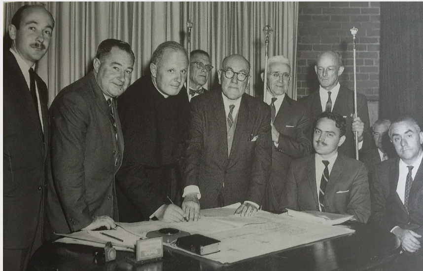
Fig. 6.9: Signing of the contract for the new church. Front row left to right: Mr Bryan Linacre, the builder Mr Gardiner, Archdeacon Codrington, architect Louis Williams, seated are architects Blyth Johnson and John Paul.
