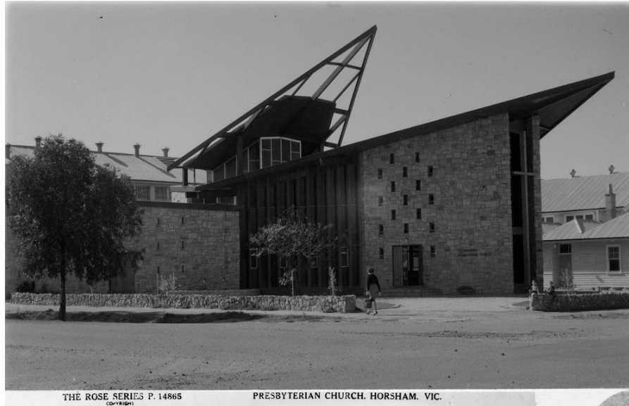
Fig. 5.43: Presbyterian Church, Horsham, Victoria, 1962 Architect: Keith Reid
