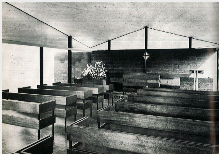
Fig. 5.53: View of the original orthogonally laid out interior.
