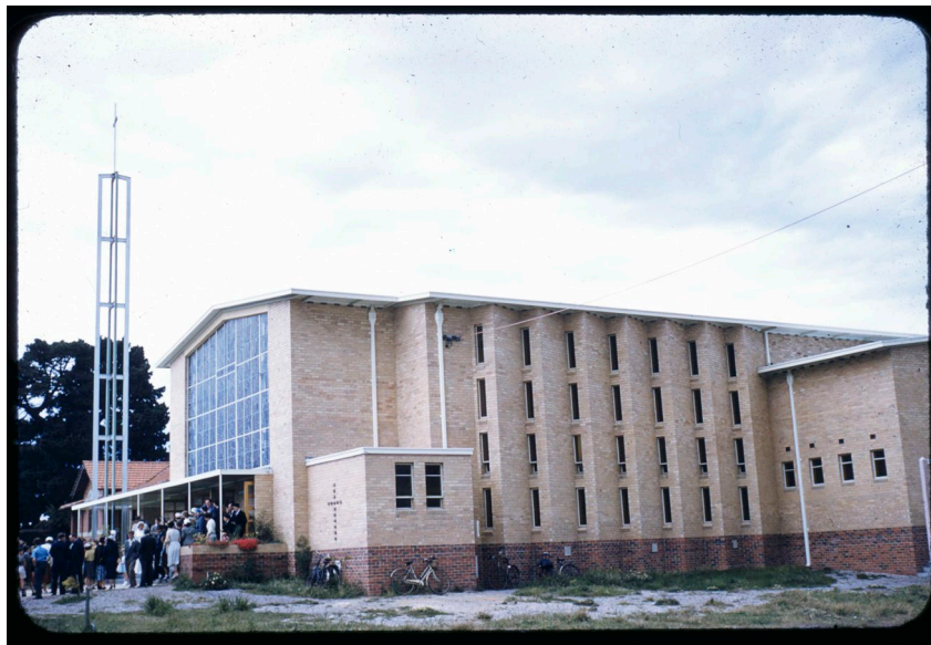
Fig. 5.1: St Francis Xavier Catholic Church, Frankston 1954 Architect: Alan G. Robertson
