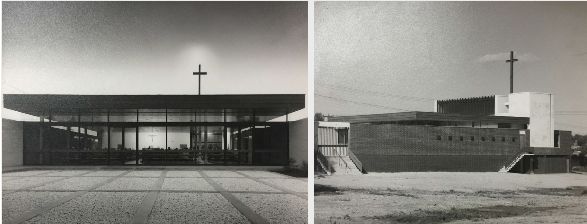
Fig. 5.61: Two views of St Joseph's Catholic Church, internal courtyard and exterior c. 1962
