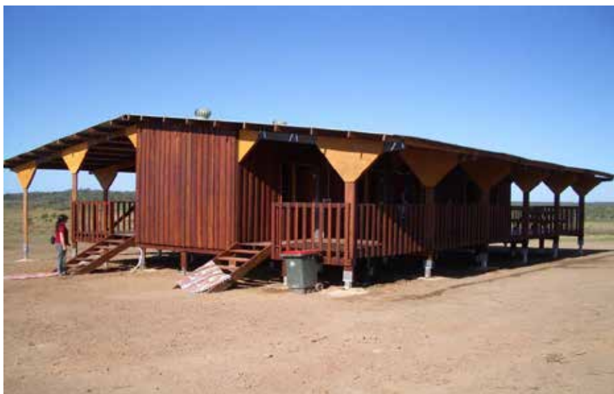
FIGURE 2 The Gumatj Bunkhouse at Garrathiya Homeland 2009. Source: Klaus Helms, CEO, Gumatj Aboriginal Corporation, 2009.
