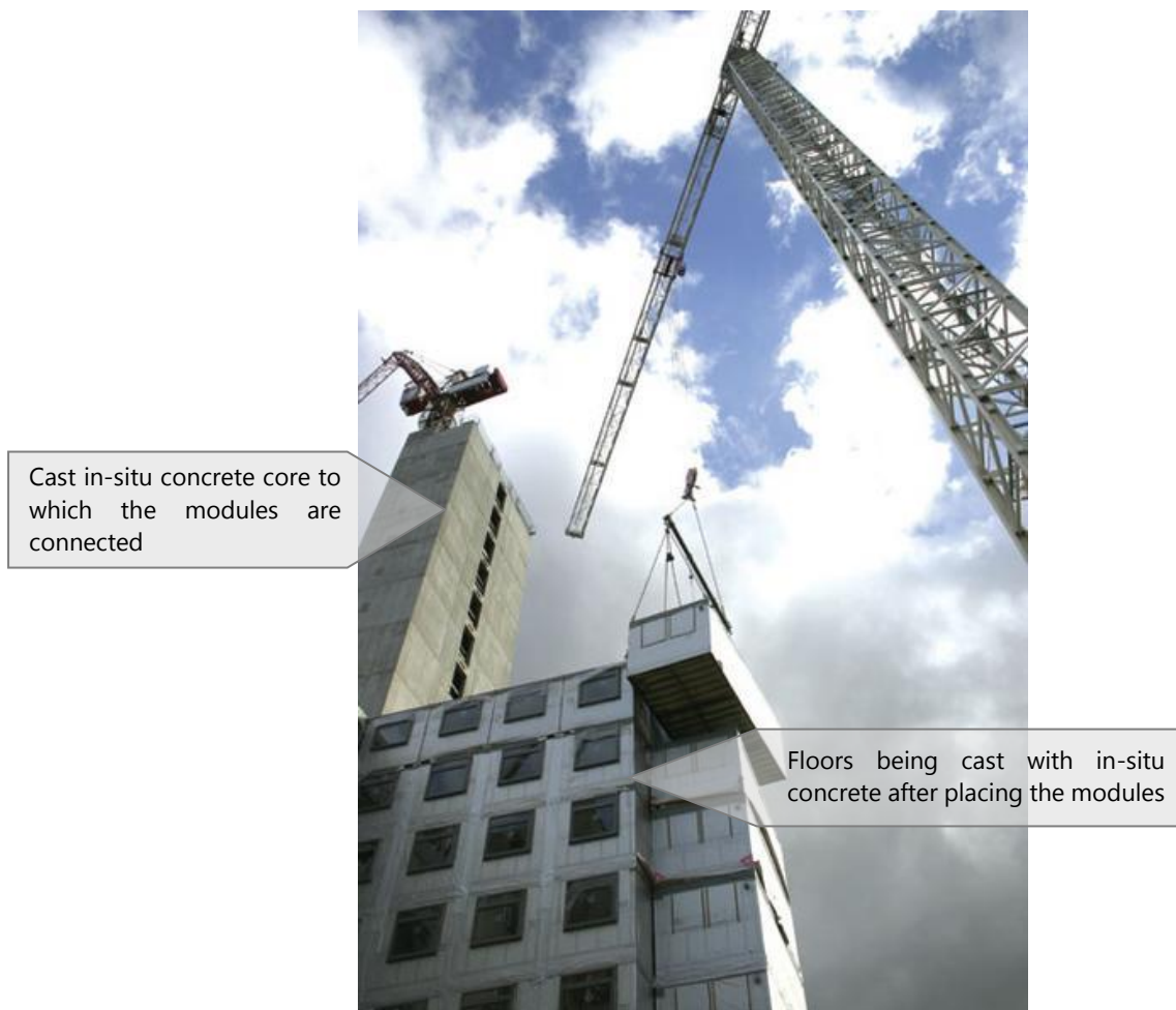
Figure 1. 7. An example of current practice in multi-storey modular construction
