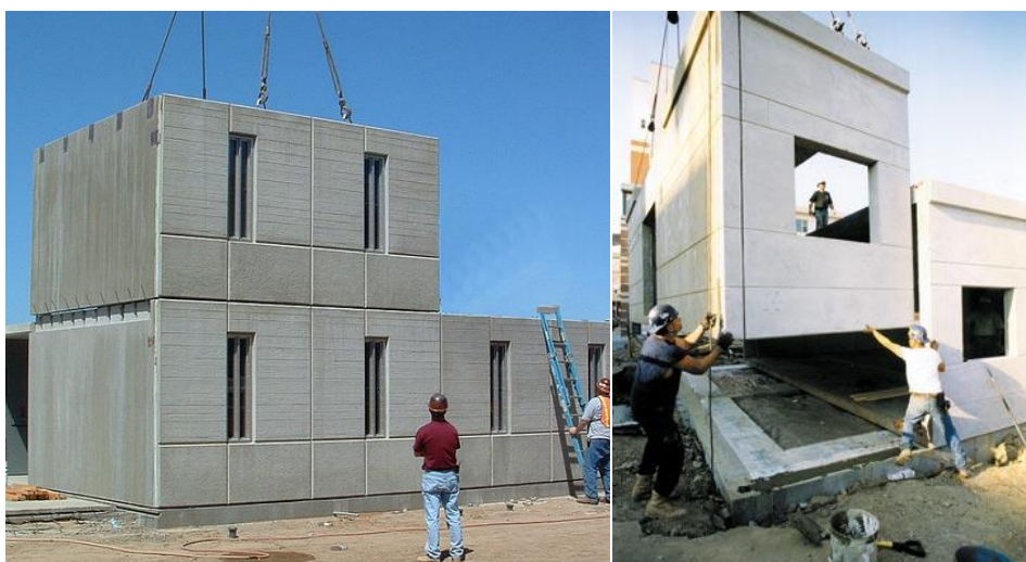
Figure 2. 3. Prefabricated modules made with concrete
