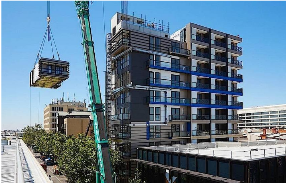
Figure 1. 6. One9 Apartments during construction (Hickory Group, 2014)
