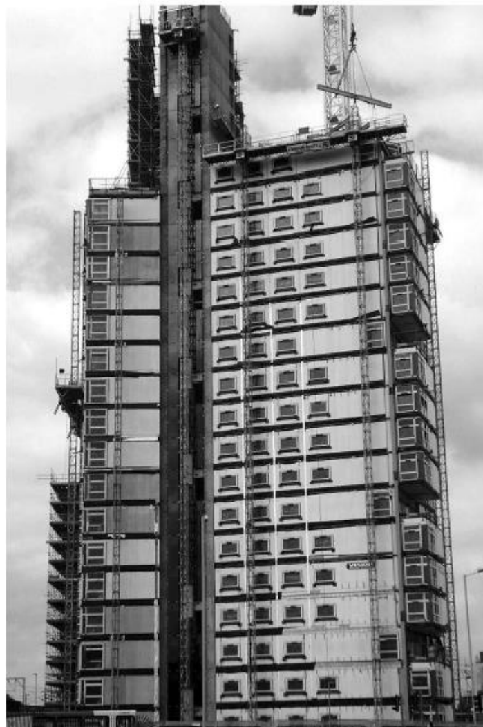
Figure 1. 4. A 25 storey modular building in Wolverhampton, UK (Lawson et al., 2012)
