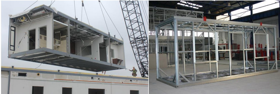
Figure 2. 4. Prefabricated modules made with steel
