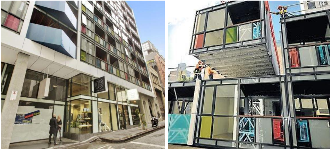
Figure 1. 2. An image from the modular building 'Little Hero' after being built and occupied (Left) and one during its on-site assembly (Right)
