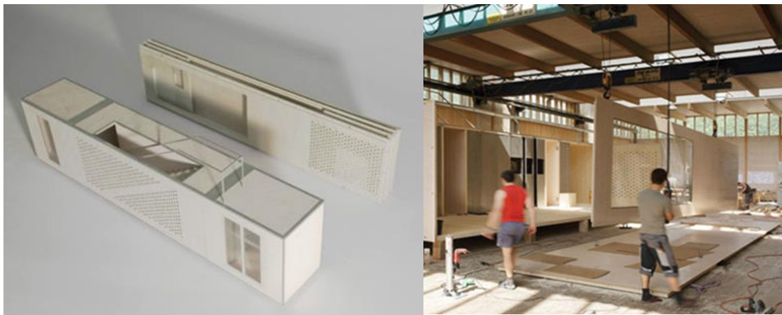
Figure 2. 2. Prefabricated modules made with timber
