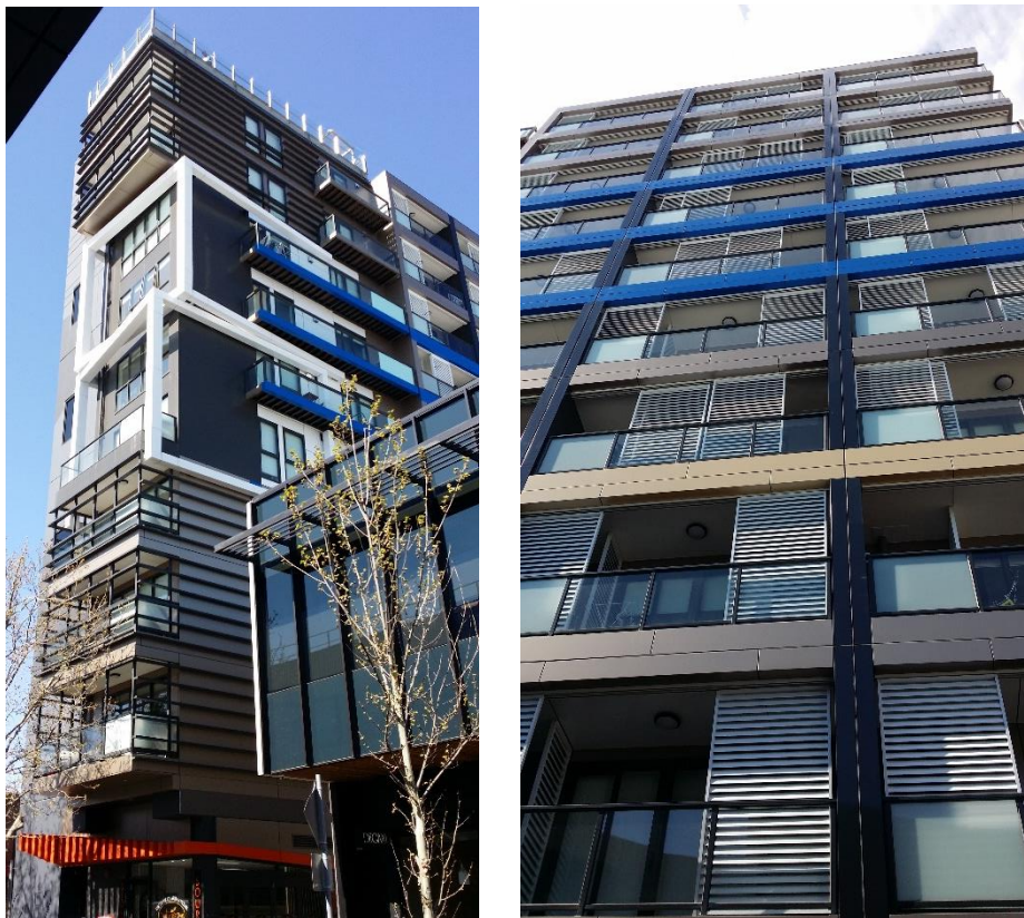
Figure 1. 5. 'One9 Apartments' modular building in Melbourne, Australia
