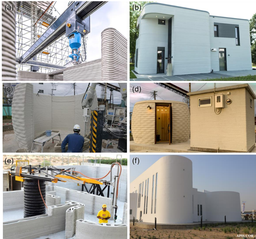
Figure 2.5. COBOD BOD 2 gantry printer (a) used to build a two-story 160 m 2 3D printed residential building in Europe (b) [18]; Cybe mobile robotic arm 3D printer (c) used to build self-contained toilet units (d) in Japan [19]; Apis-cor printers in polar coordinates (e) used to build a two-story 640 m 2 world largest 3D printed building (f) [20].
