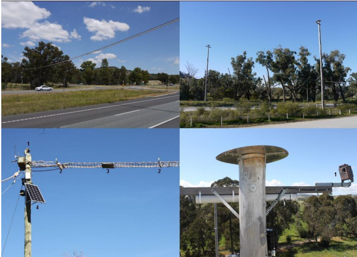
541 Figure 2. Canopy bridges (top left) and glider poles (top right) along the Hume Freeway in 542 south-east Australia. Monitoring equipment (bottom left and right) included motion-triggered 543 cameras (1), active-infrared sensors (2), PIT tag antennae (3) and power supply (4).
