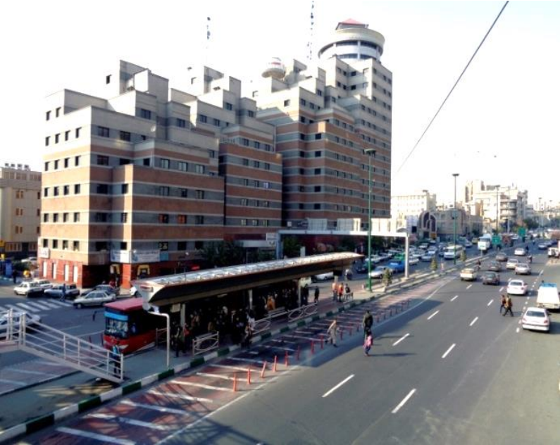
Figure 10.3. BRT station along the Navab Highway with partially dedicated lanes and wider station spacing
