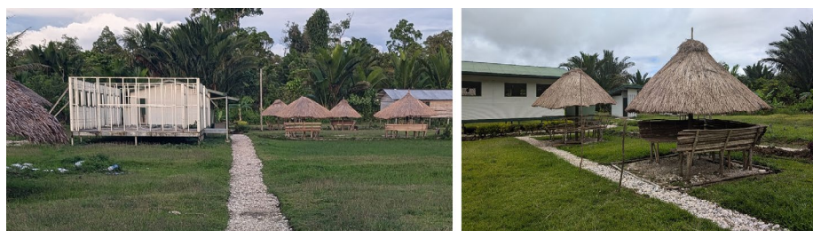
FIGURE 3 Photos of small, thatched lunch shelters and pathways of white stones constructed by volunteer labour at Soabi Primary School.
