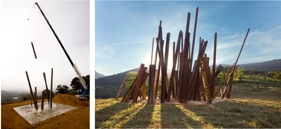
Figure 41 Left image: Chris Burden's Beam Drop action sculpture in the making. Right image: The completed beam sculpture in the hardened concrete. Image courtesy: Instituto Inhotim, Brazil © Eduardo Eckenfels, 2013.
