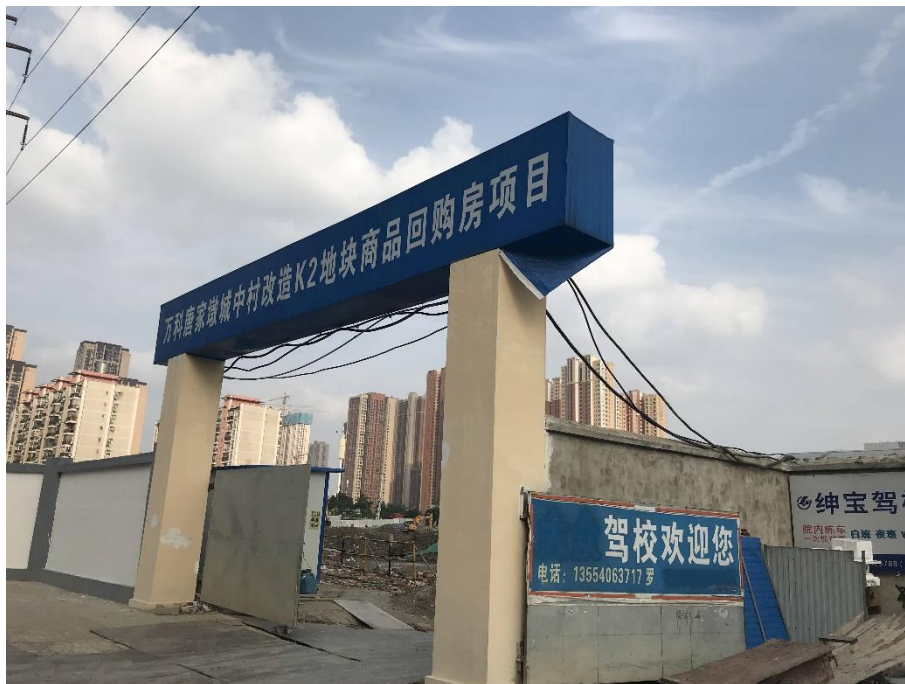
Figure 6-13. An urban village renovation project on the northside of Hankou Railway Station
