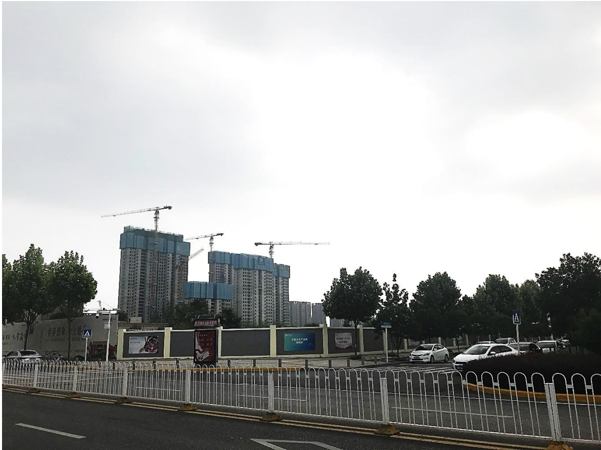
Figure 5-9. Residential buildings under construction in front of the West Station Square
