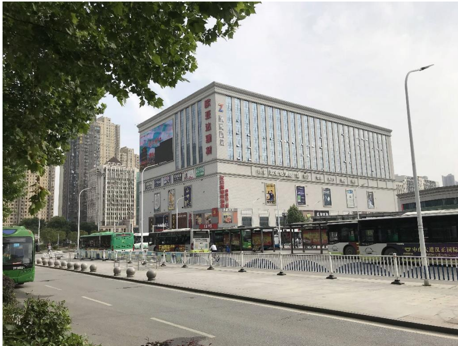
Figure 6-15. OUYAD Plaza (developed by Tianfeng) and the separate bus station
