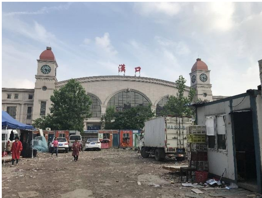
Figure 6-12. Undeveloped North Station Square of Hankou Railway Station
