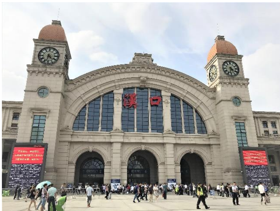
Figure 6-1. Hankou Railway Station (Exterior)
