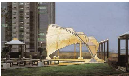
Fig.12: This fabric membrane structure at the Hyatt Regency in Osaka uses a photocatalytic clear coat based on \text{TiO}_2 , which creates antibacterial effect. (Ashby et al. , 2009)
