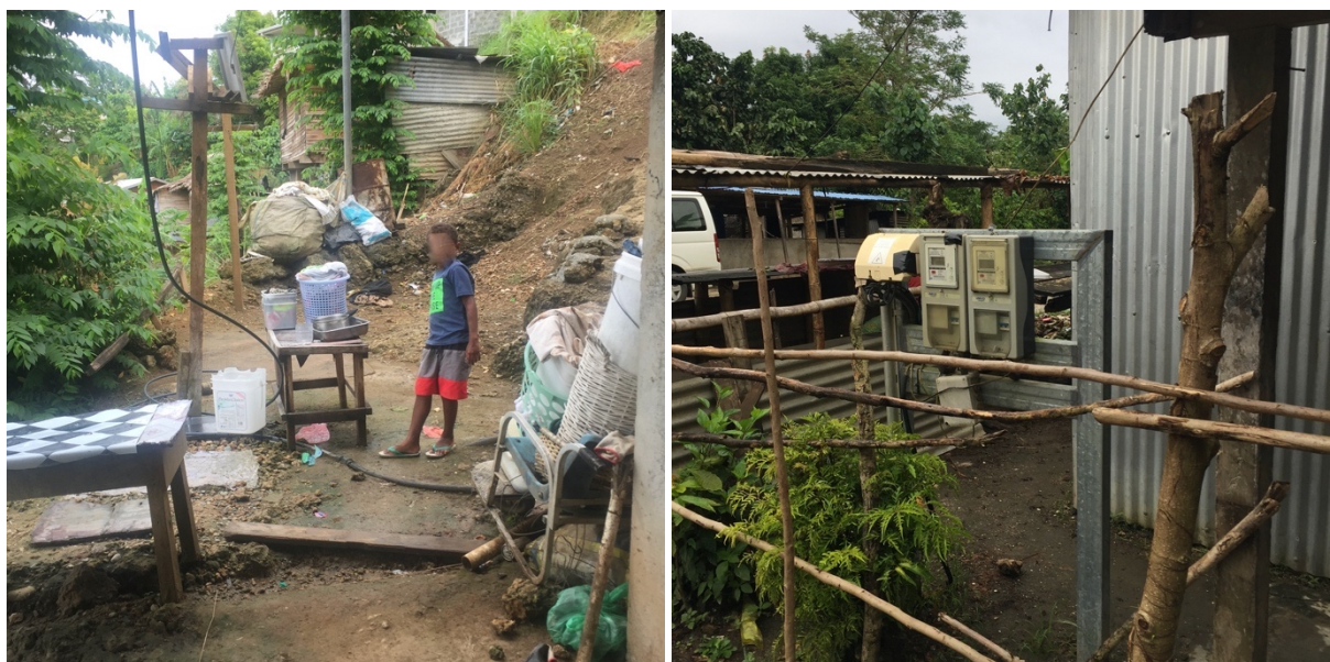
FIGURE 7.7: SHARED WASHING FACILITIES, HONIARA & A SHARED METER, PORT VILA
