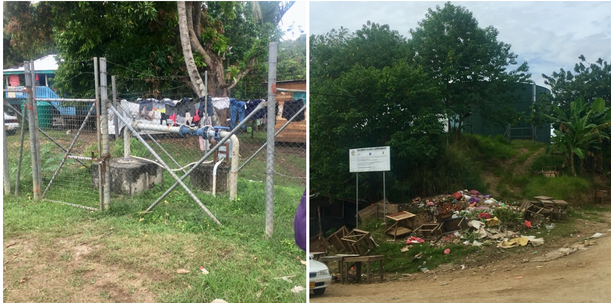
FIGURE 8.2: SOLOMON WATER BOREHOLE ACCESS POINT, JABROS COMMUNITY (LEFT) & URBAN STORAGE TANK AT THE NEARBY TOWN BOUNDARY IN GILBERT CAMP (RIGHT)
