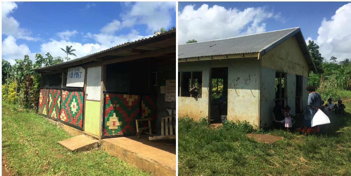
FIGURE 6.12: INFORMAL SHOP (LEFT) & COMMUNITY HALL (RIGHT) IN ETAS, PORT VILA
