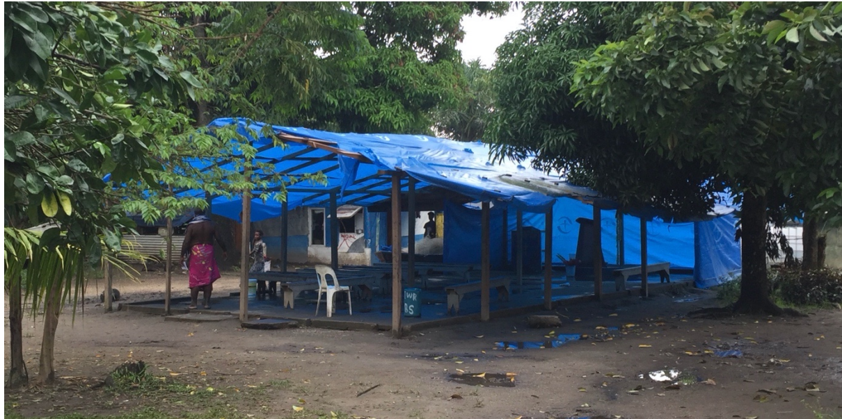
FIGURE 7.4: WILLIE ROMA CHURCH BUILDING, BLACKSANDS COMMUNITY, PORT VILA
