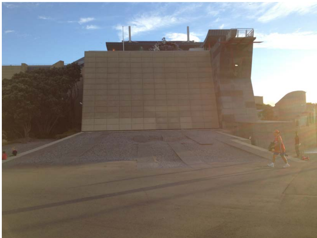
Figure 5.11. Author's photograph, The isolated waka landing ramps at Te Marae, Te Papa , 2013.
