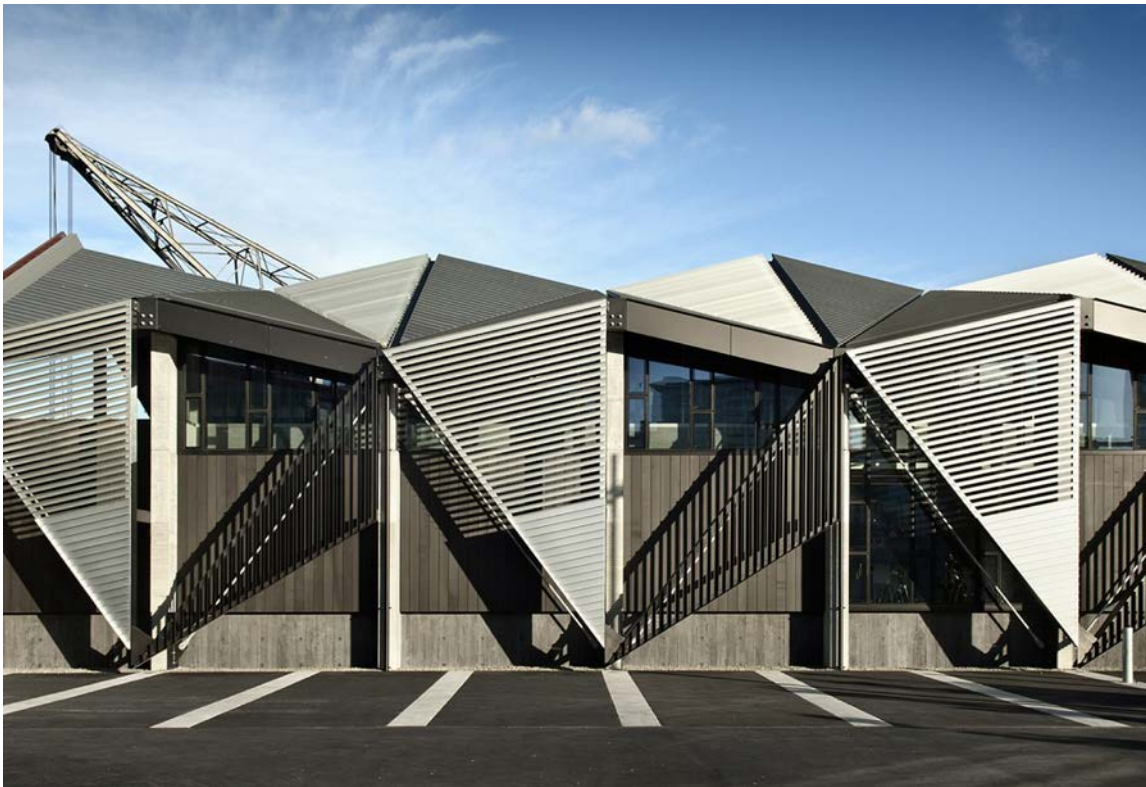
Figure 6.14. Architecture+. Te Wharewaka , Architecture Plus Ltd, http://architectureplus.co.nz/public/wharewaka/ .
