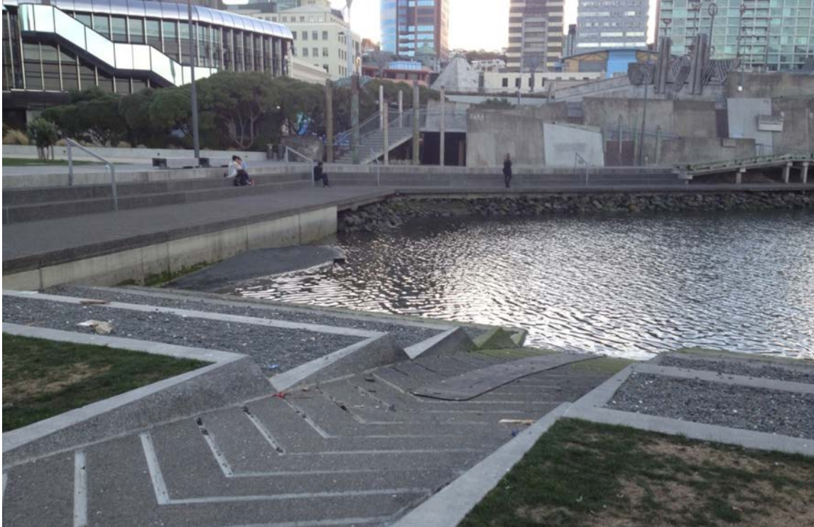
Figure 6.13. Author's photograph, The waka ramps continue the patterning of Te Wharewaka, and lead into the new lagoon, 2014.
