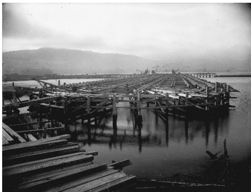
Figure 2.38. Sydney Charles Smith, Graving dock under construction, Wellington harbour, 1909 , '1888-1972: Photographs of New Zealand', Ref: 1/1-019641-G. Alexander Turnbull Library, Wellington, New Zealand. http://natlib.govt.nz/records/22416460
